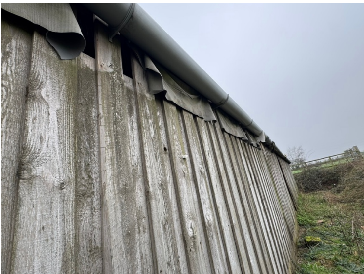
Photo 5: B1 exterior, showing same wall as Photo 4.
