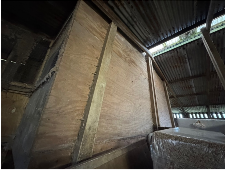
Photo 1: External wall of chicken house (whole structure lies within B1)
