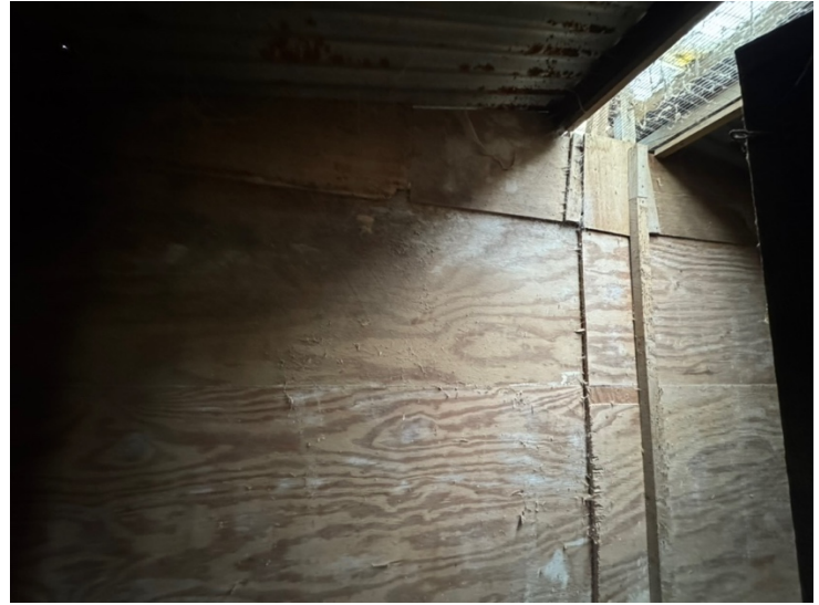
Photo 2: Internal portion of chicken house showing well-sealed, single skinned plywood
