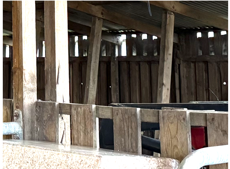
Photo 4: Building B1 interior wall
