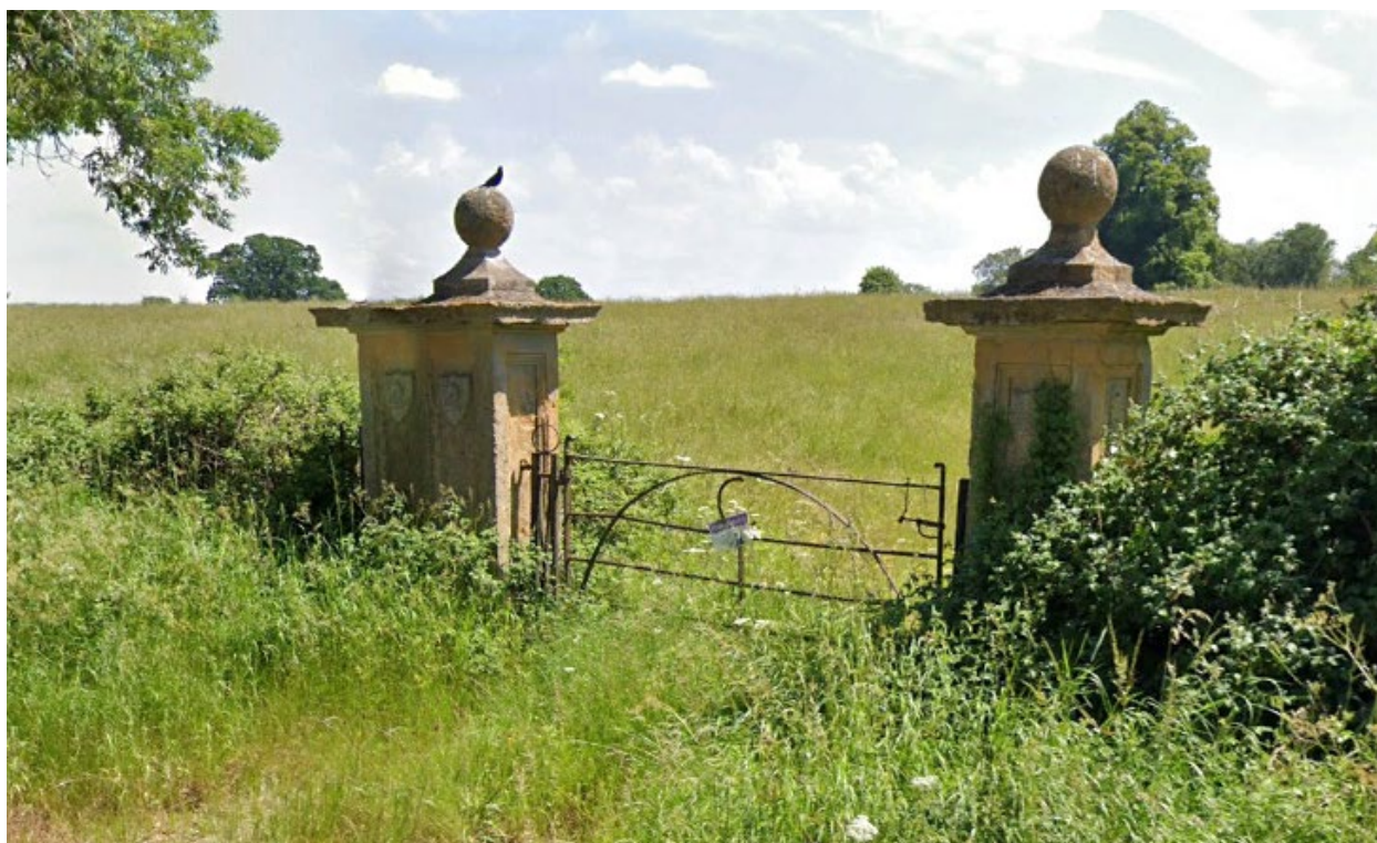
Stone gate piers to the carriageway to the former Orton Hall, looking south (© Google Earth)
