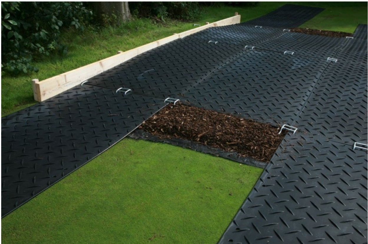
Image 1 – Ground-Guards temporary tree root protection - example
