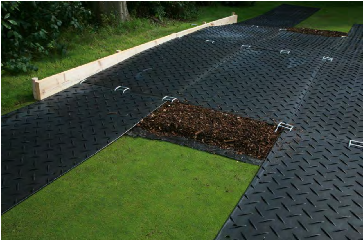
Image 1 – Ground-Guards temporary tree root protection - example
