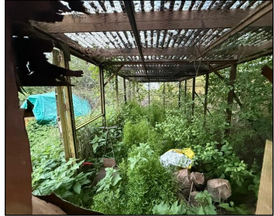
Photograph 8: Extension built onto the eastern elevation of Building B1. Photograph taken facing east.
