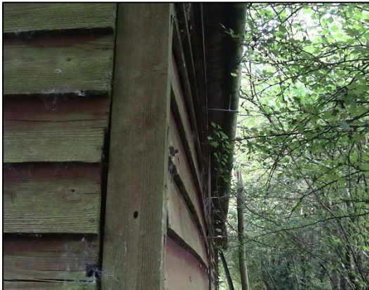
Photograph 3: The eastern elevation of Building B2. Photograph taken facing north.
