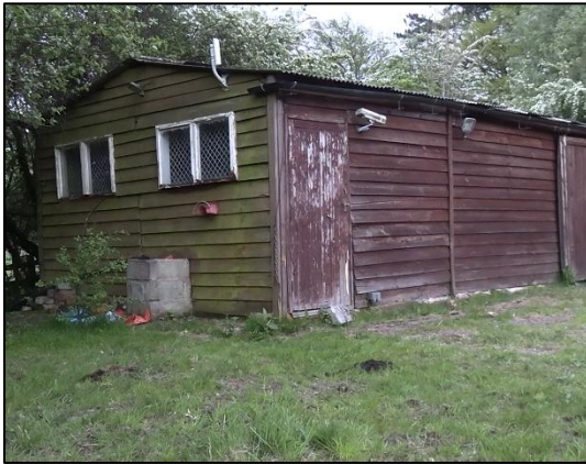
Photograph 1: The northern and western elevation of Building B2. Photograph taken facing south.
