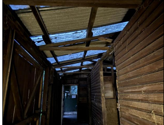
Photograph 4: The internal area of Building B2. Photograph taken facing north.
