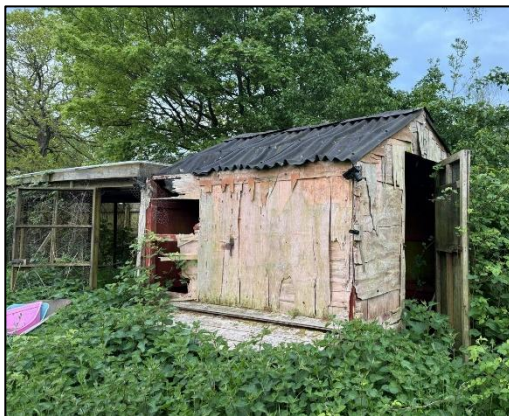
Photograph 5: The northern and western elevation of Building B1.
