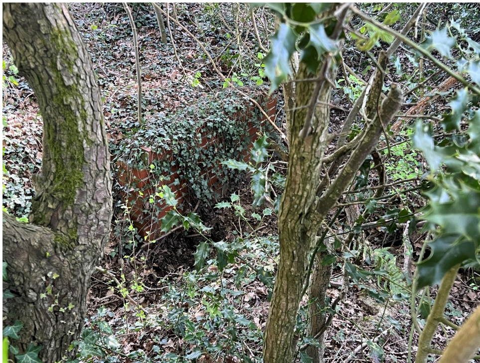
Photo 1. Existing Hedwall – North-Eastern Outlet
