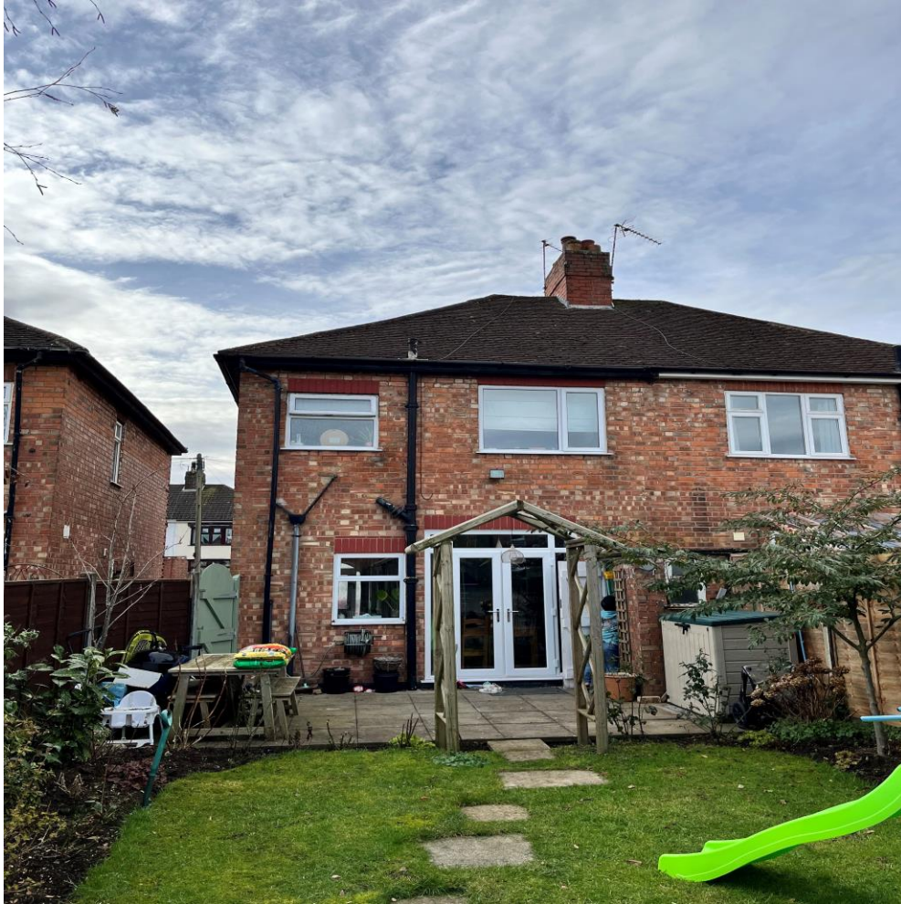
Photograph 2. The Rear Elevation
