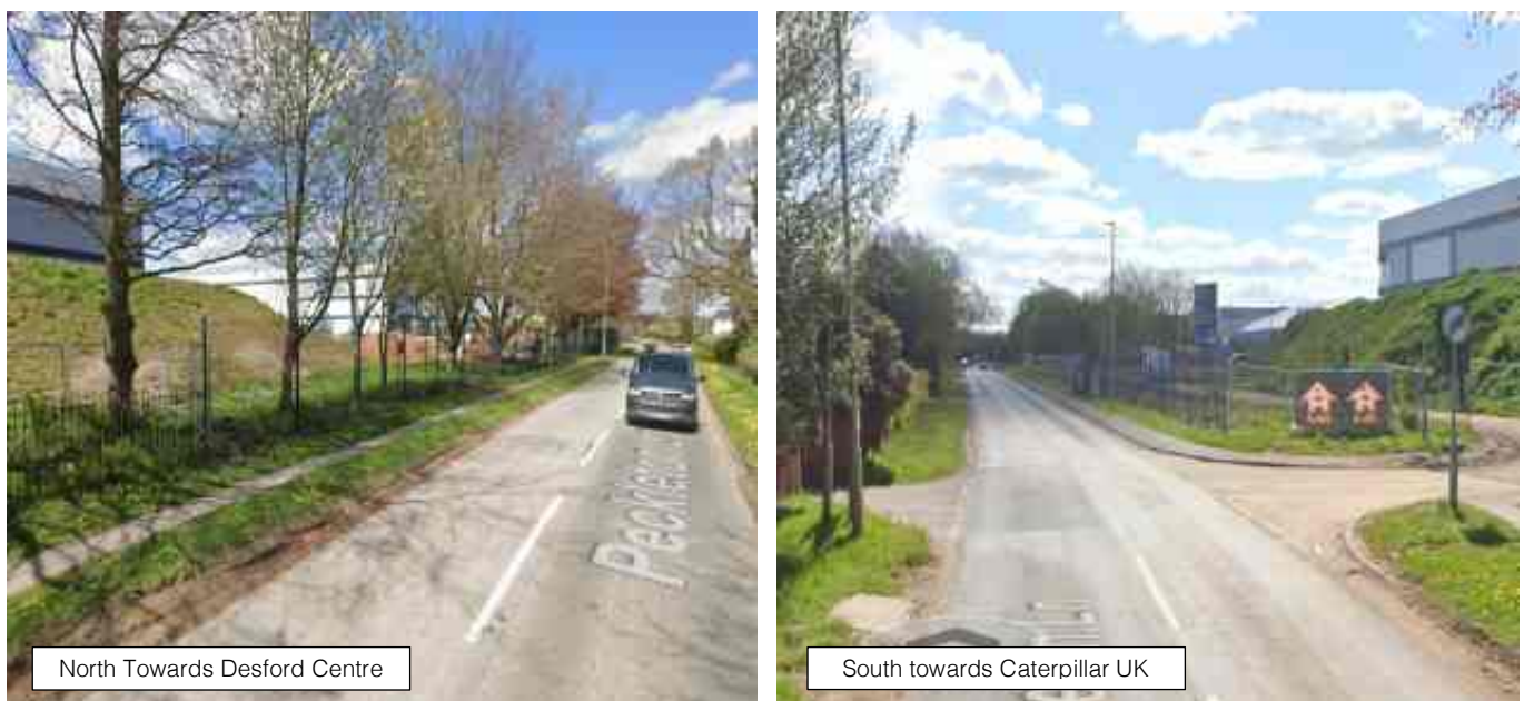
Figure 4.2 Footway Provision along Peckleton Lane
