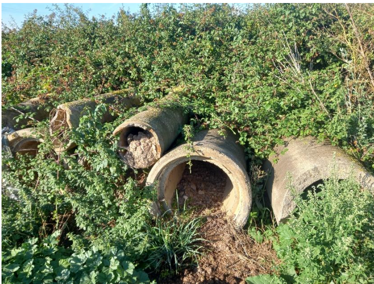
Picture 7 – View of a concrete pipes in the center of Area 1 next to manure pile
