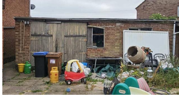
West elevation of B2
