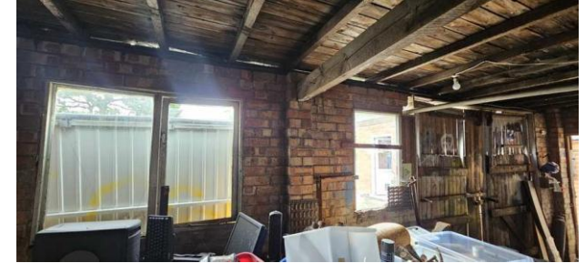
Interior of building B2
