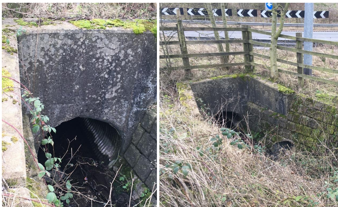
Figure 3.7: Soar Brook (M69/A5) Culvert (Taken During Site Visit – 04/03/20)
