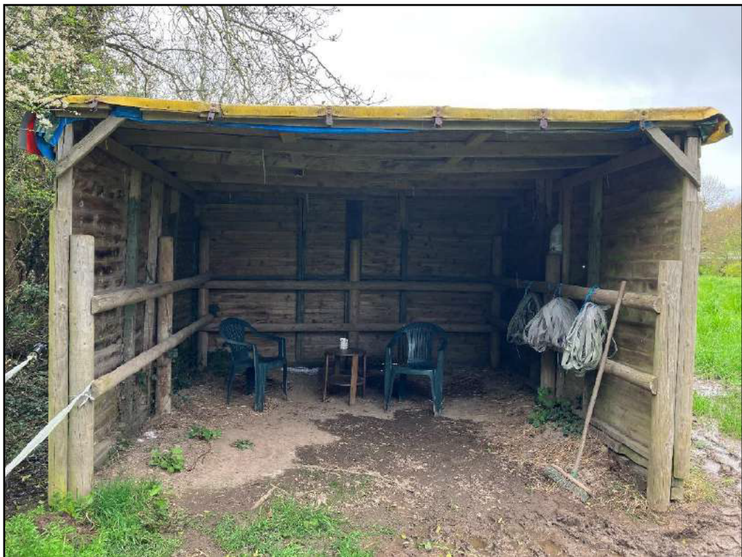
Figure 8: Building B2 on site
