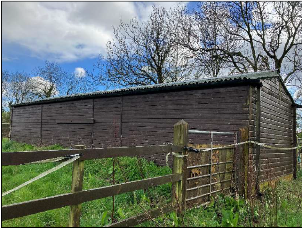
Figure 7: Building B1 on site
