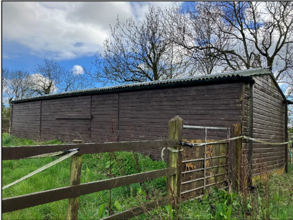
Figure 7a. Building 1 on site.
