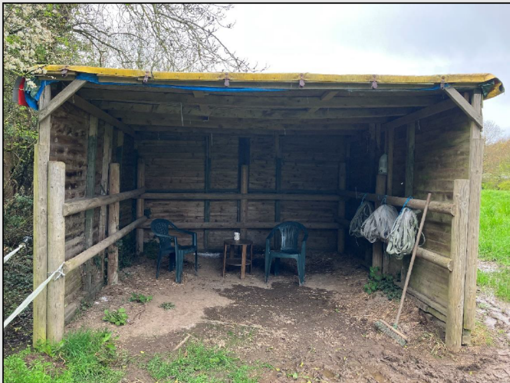
Figure 7b. Building 2 on site.
