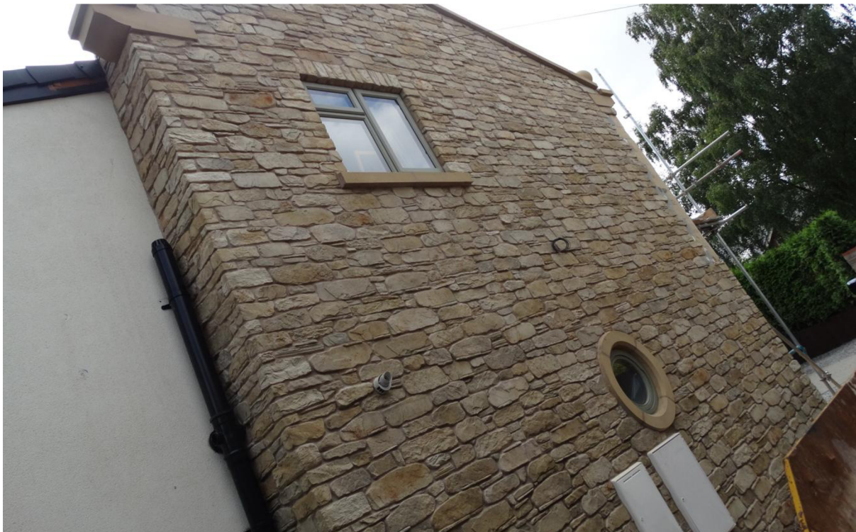
Image 4 – West facing elevation of the property where the proposed works will take place
