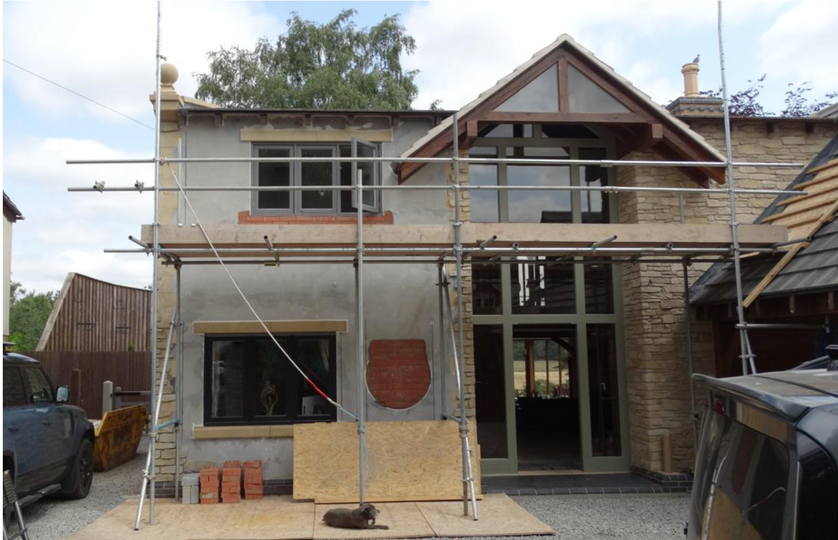
Image 1 – South facing elevation of the property
