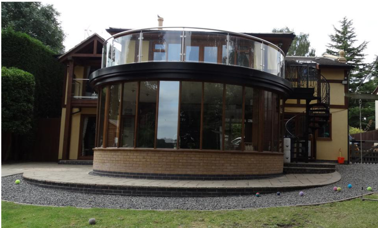
Image 2 - North facing elevation of the property
