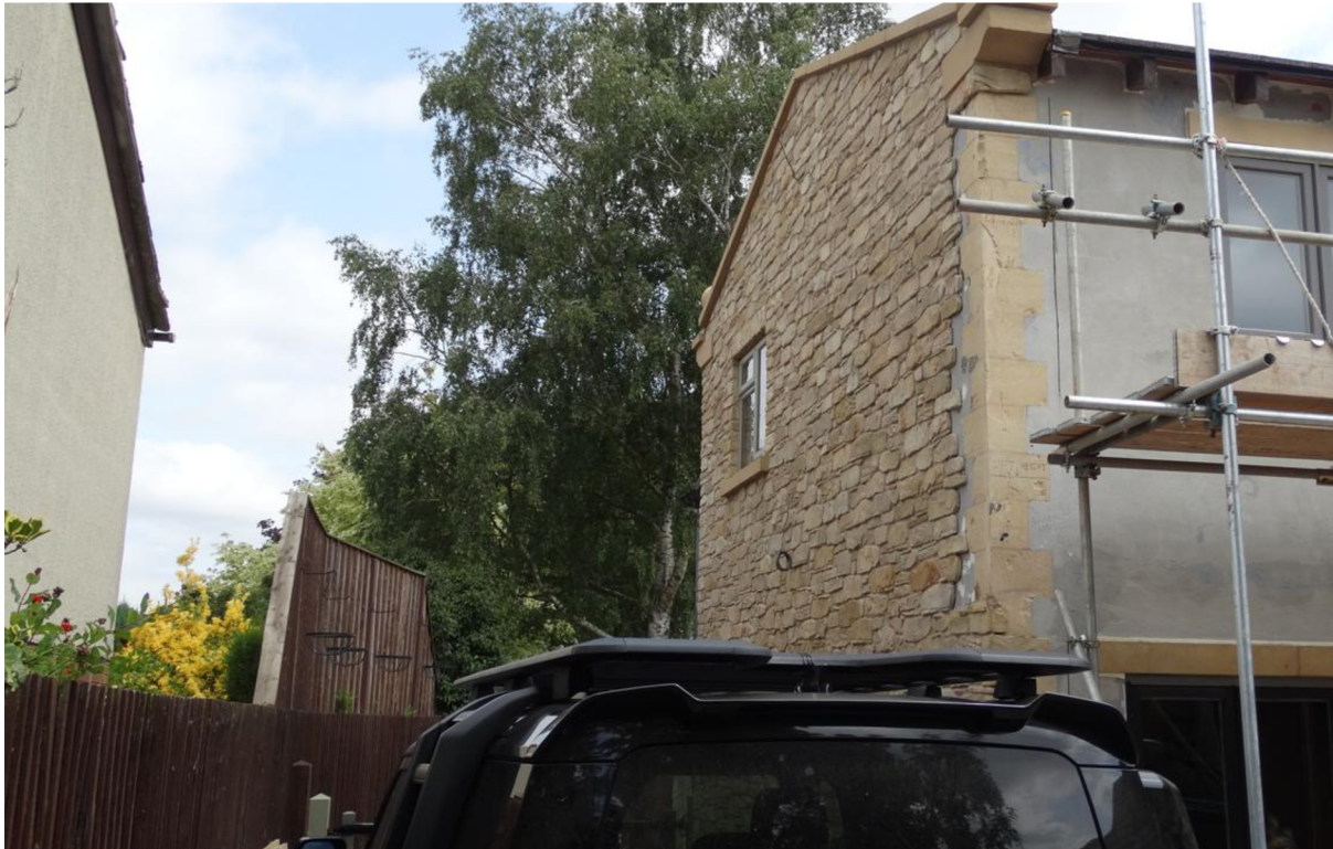
Image 3 – West facing elevation of the property where the proposed works will take place
