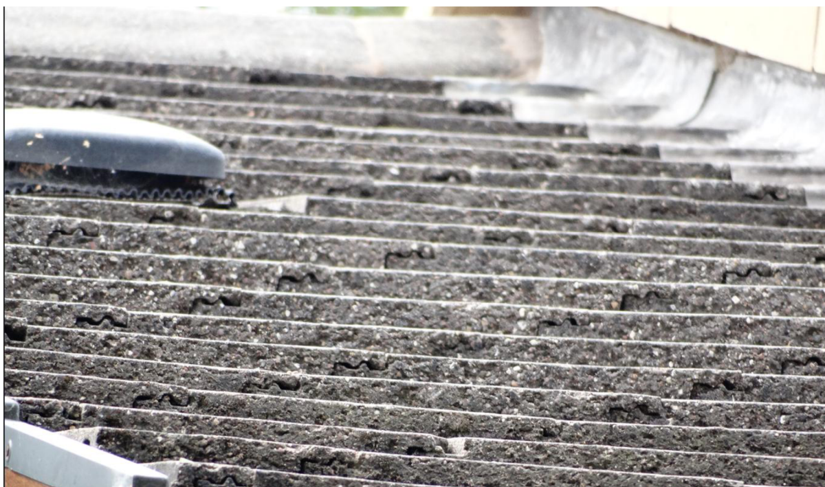
Image 5 – Example image of tiled roof coverings above the West section of the property
