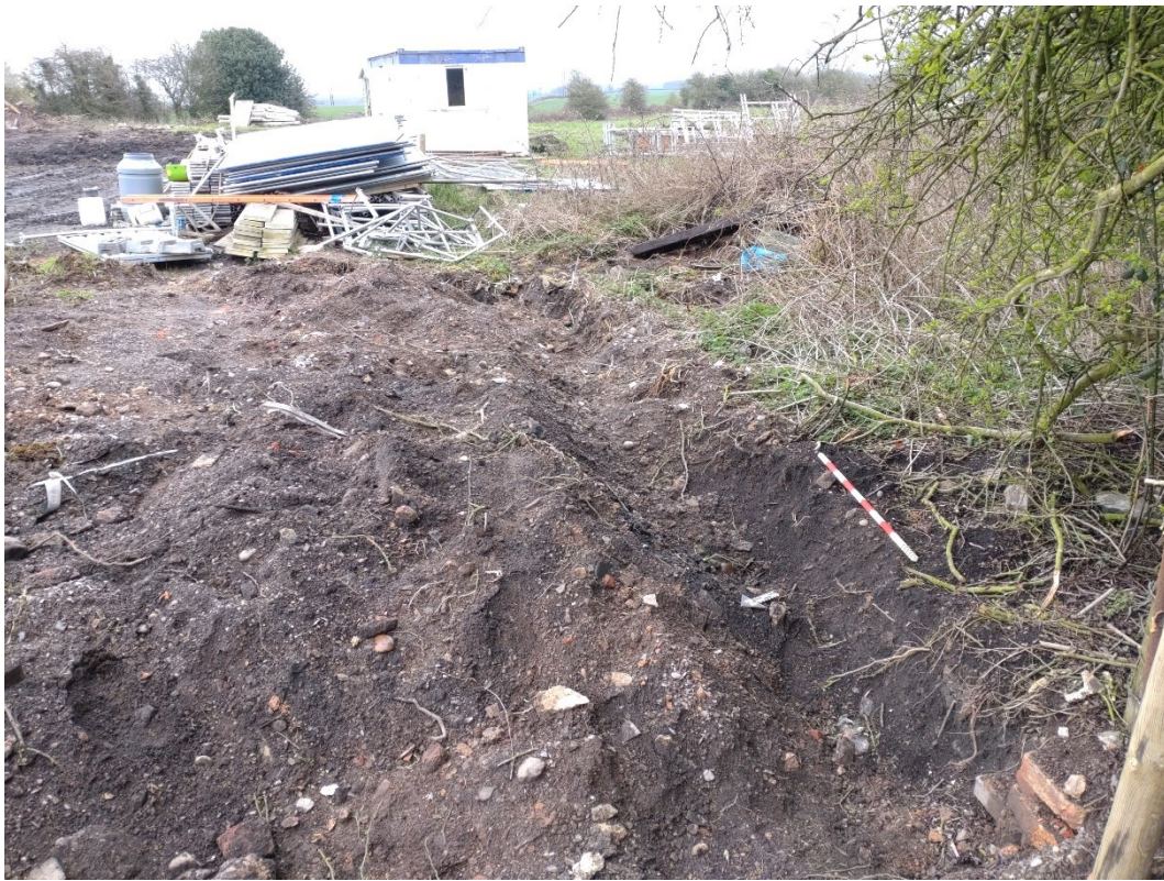
Figure 12: Location of demolished dry stone wall, looking south-east, 1m scale.
