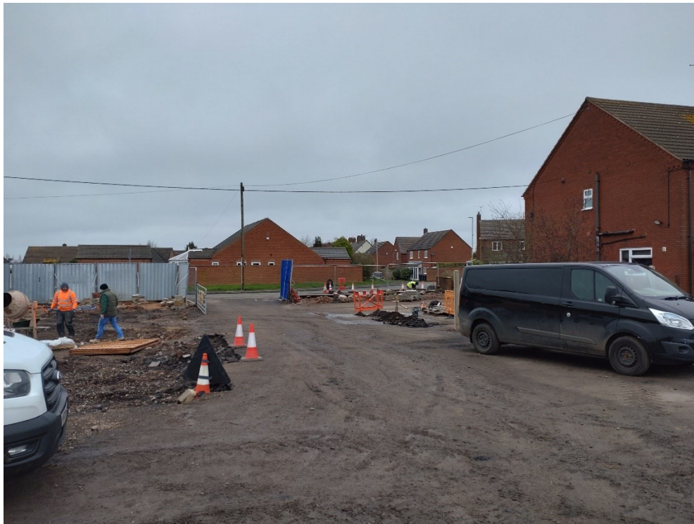
Figure 4: Pre-groundworks, looking north across the site
