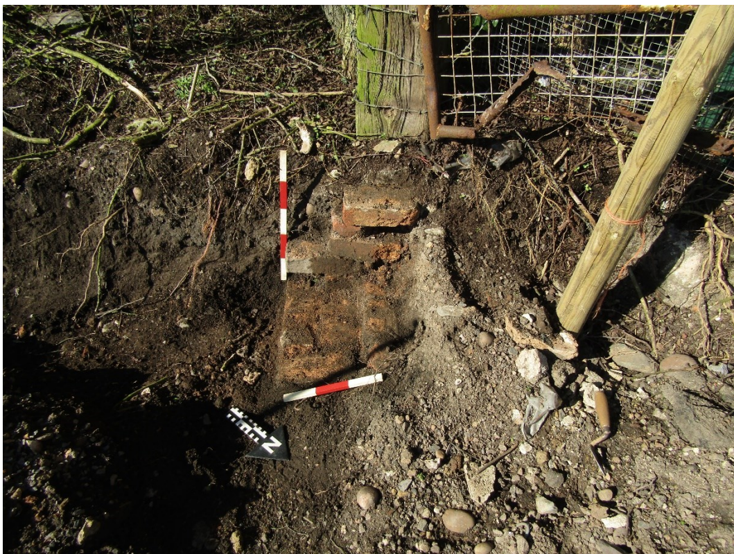
Figure 13: In situ brick foundation towards north of demolished dry stone wall, looking south-west, 0.30m x 0.50m scale.
