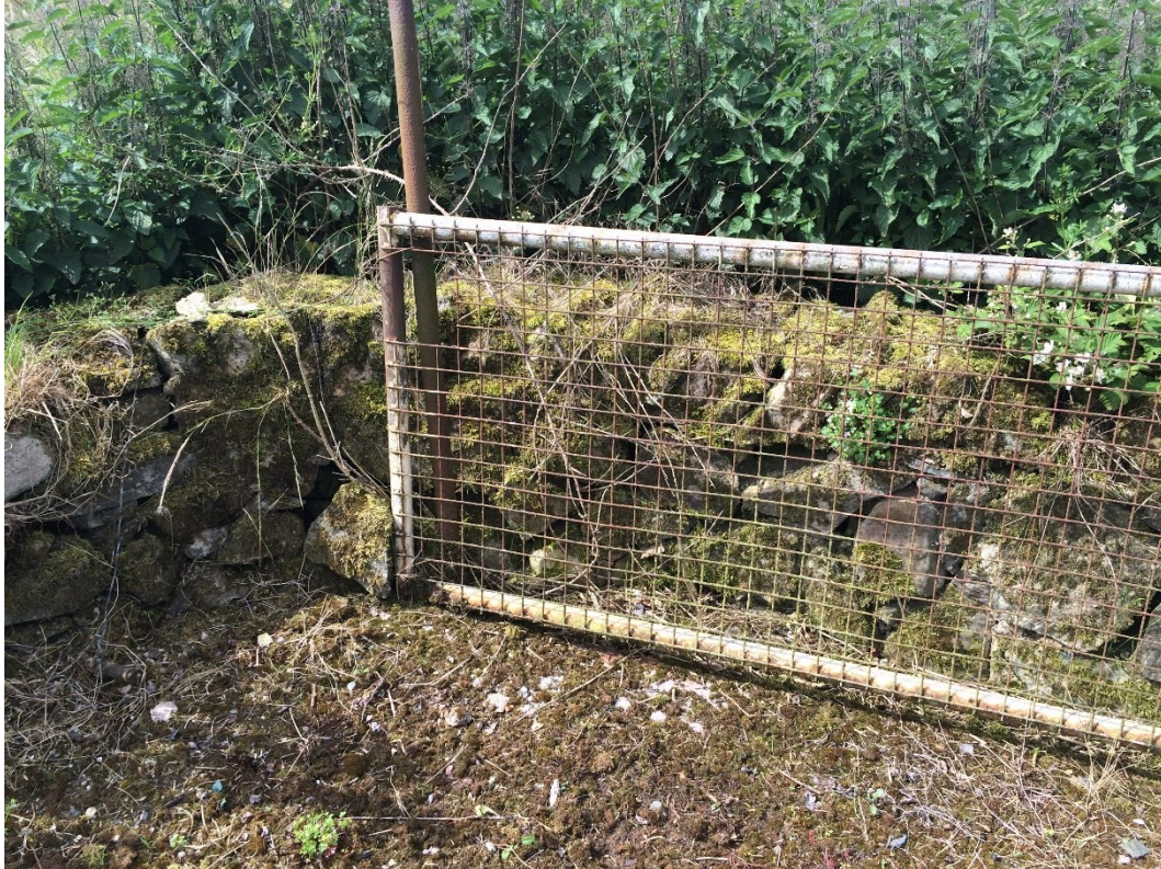
Figure 10: Close up of dry-stone wall, looking south-west (Brown 2016).
