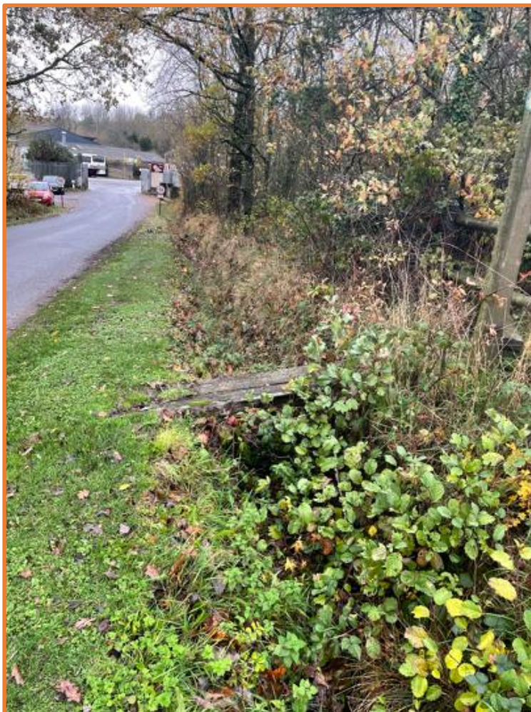
Figure 1: View northwest showing ditch towards existing industrial estate
