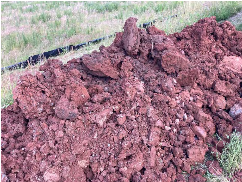
Trial Pitting (Embankment) note unconsolidated material
