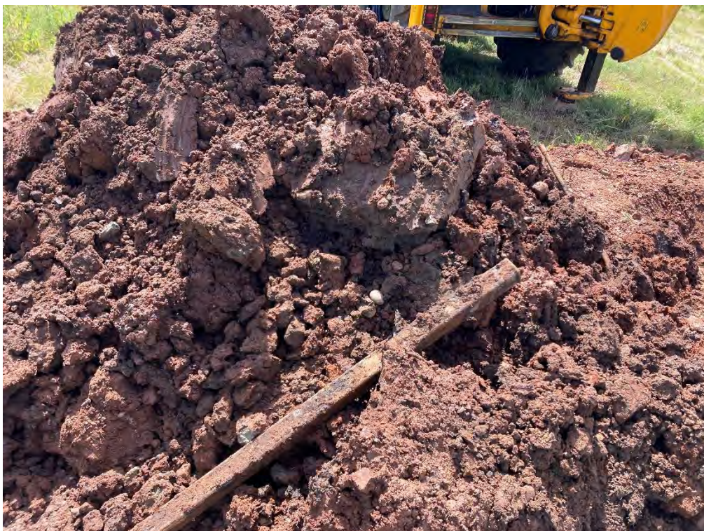
Trial Pitting (Embankment) note rare anthropogenic material
