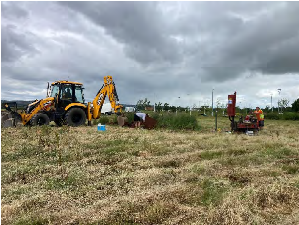
Trial Pitting and Window Sampling
