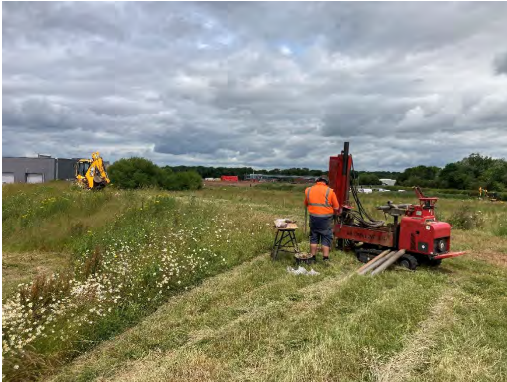
Window Sampling (embankment)
