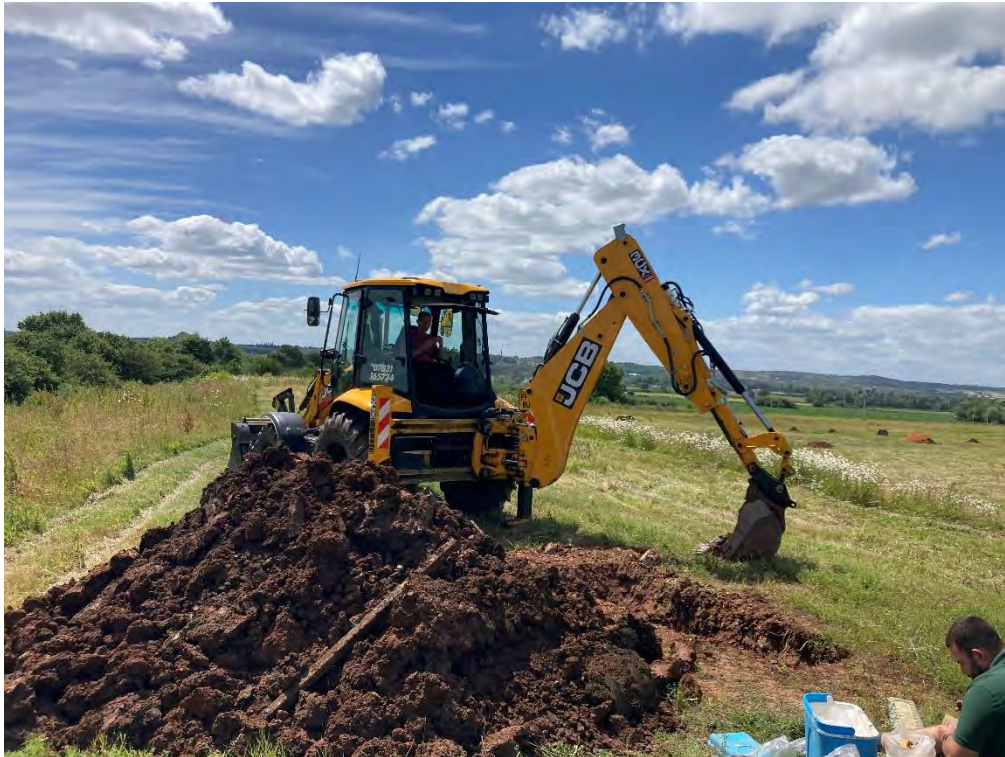
Trial Pitting (Embankment)
