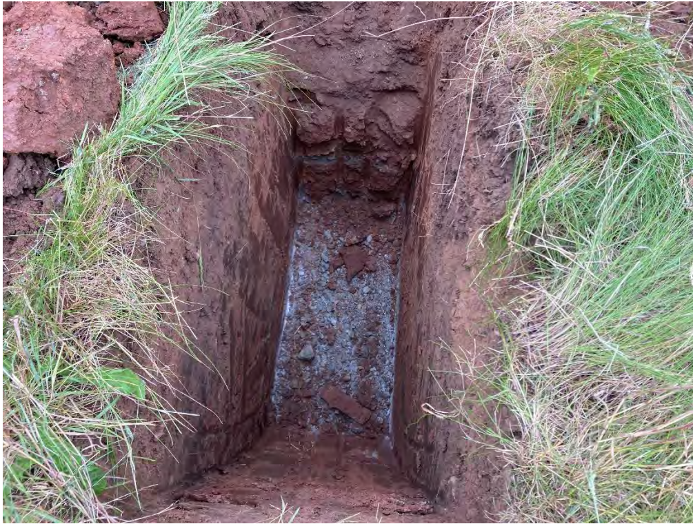
Trial Pitting note refusal on rock quality strata
