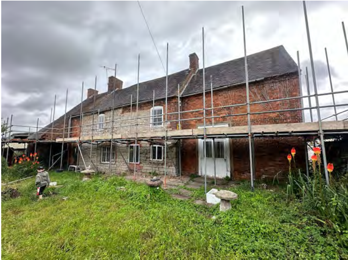
Plate 3: Western elevation looking north-east
