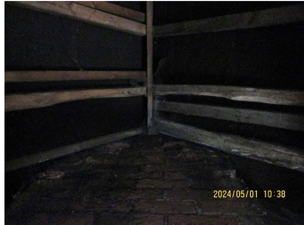
Exposed ridge and felt lining
