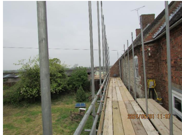
Western elevation from scaffold
