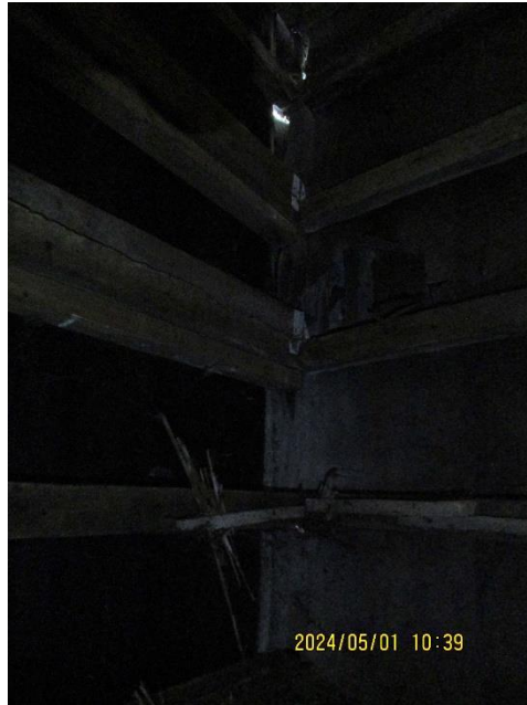
Daylight visible from within the roof space
