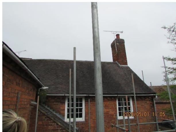
Southern view of eastern projection from scaffolding
