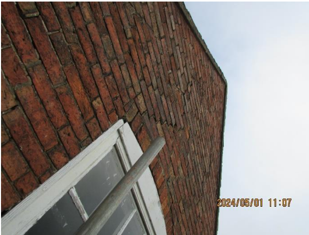
Southern gable wall from scaffold
