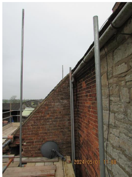
Lean-to viewed from scaffold
