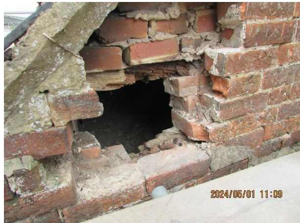
Access into lean-to void
