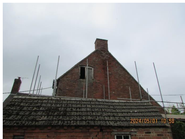
Northern gable end with lean-to
