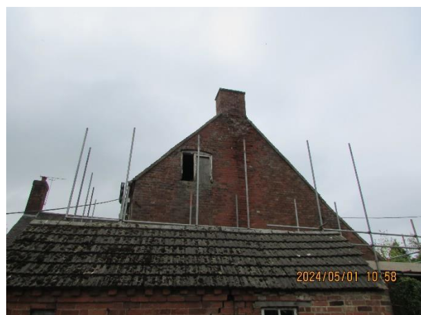
Northern gable end with lean-to
