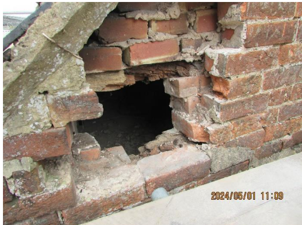
Access into lean-to void
