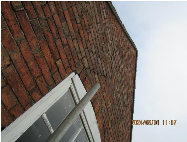
Southern gable wall from scaffold
