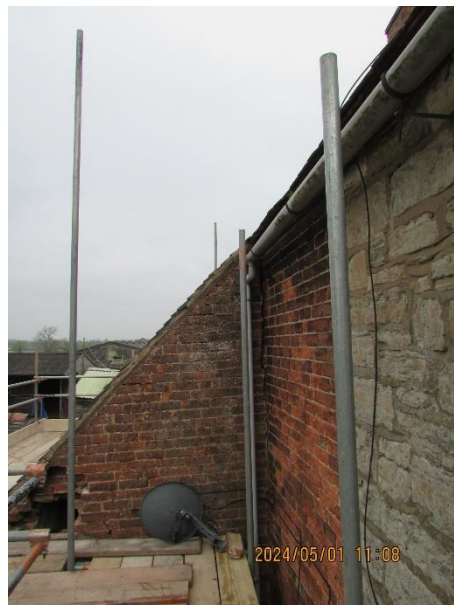
Lean-to view from scaffold
