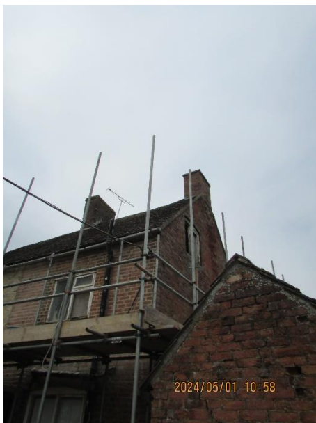
Northern gable end
