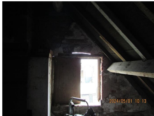
Open window northern gable
