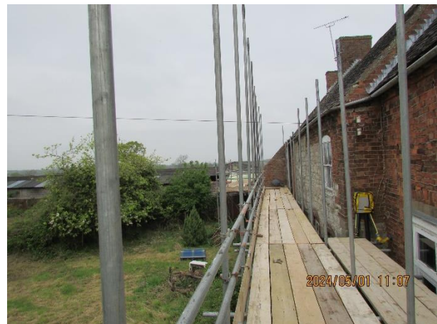
Western elevation from scaffold
