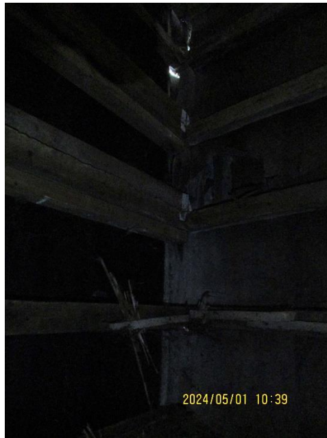
Daylight visible from within the roof space
