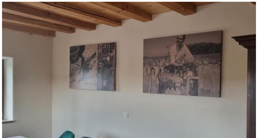
EXAMPLES OF INFRARED PANEL HEATERS AS INSTALLED.
