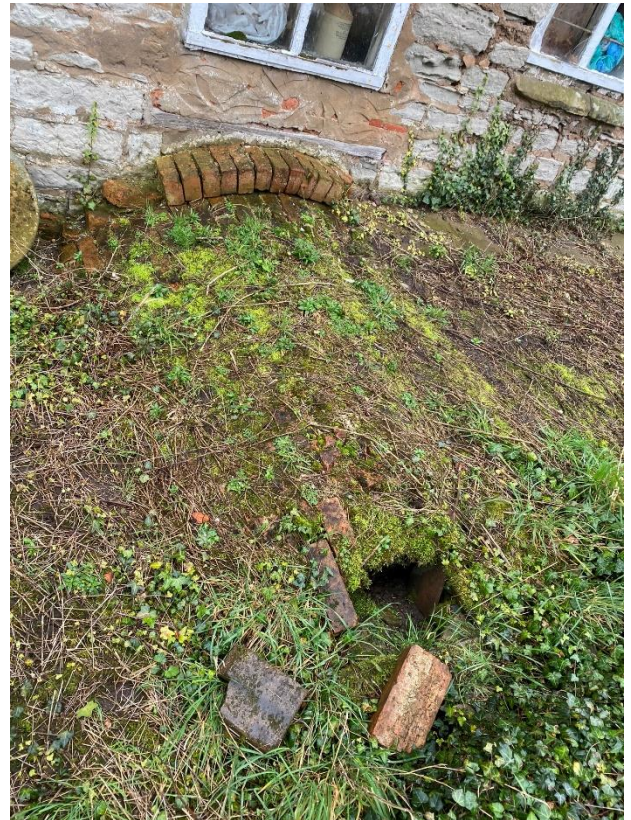
Archway access to basement
