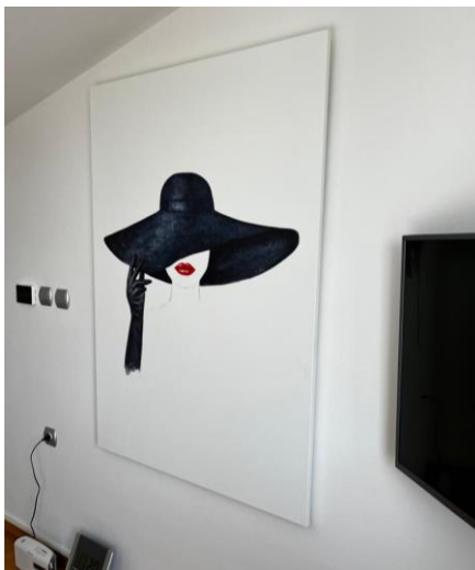
EXAMPLES OF INFRARED PANEL HEATERS AS INSTALLED.
