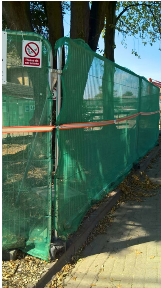
Photograph 6 (Example of tree protection barriers placed adjacent to hard surface &/or temporary ground cover)
