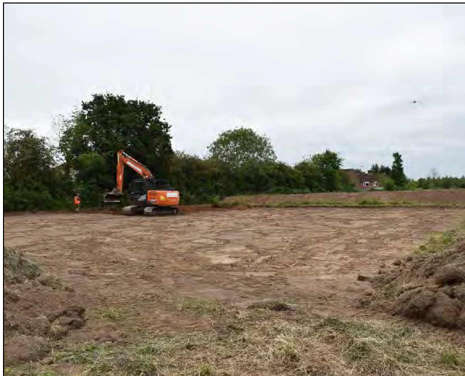
Plate 1: Site prior to subsoil stripping looking SW
