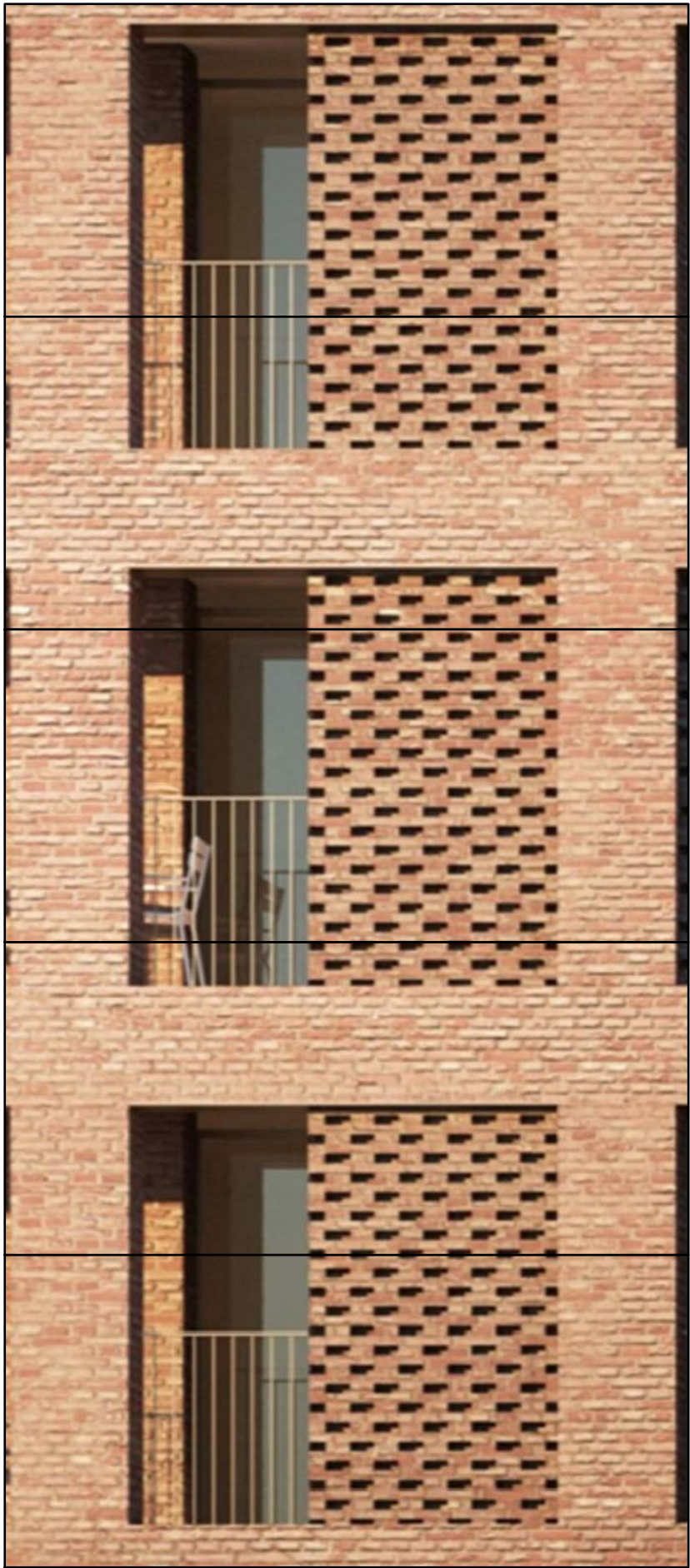
Rear elevation hit and miss brickwork screening 3.75 Metres to the rear of the habitable room windows
