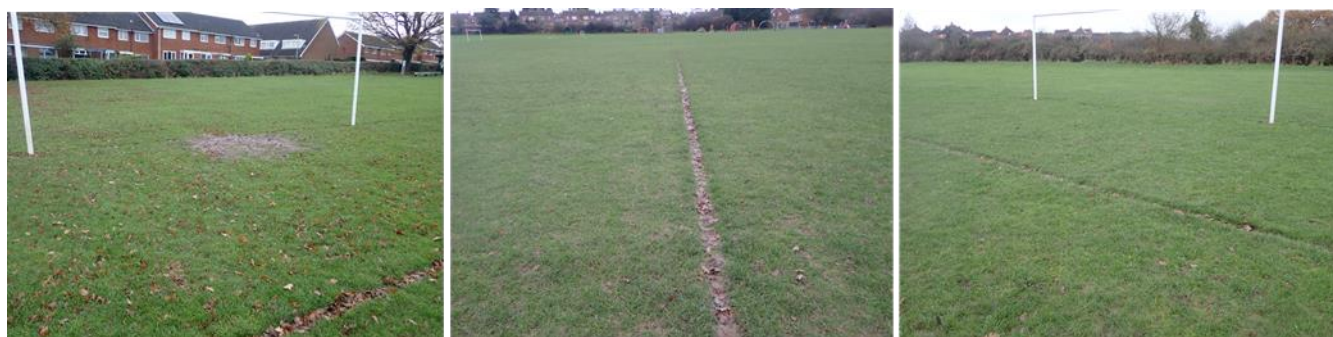
Figure 3-8 Ground cover in key areas on F2
