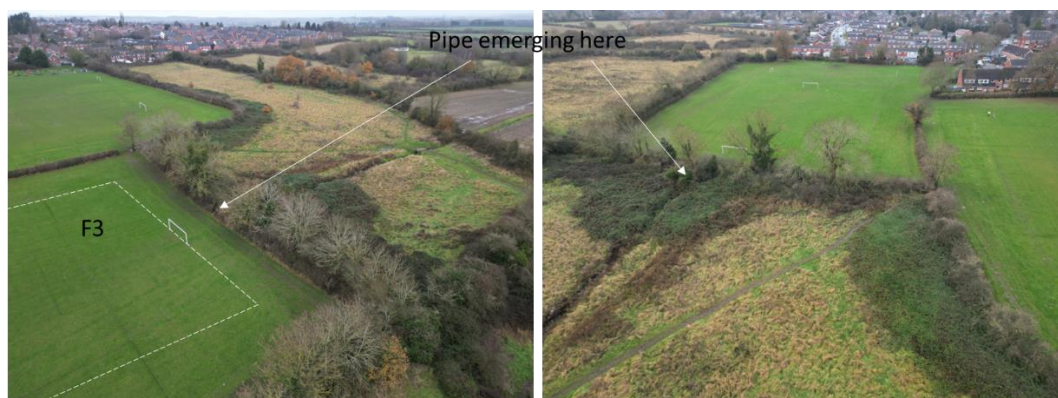
Figure 3-11 Point of emergence of culverted stream
