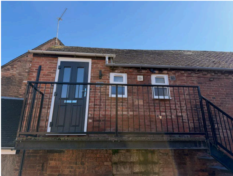
Fig 4. Flat 5A obscured windows and door
