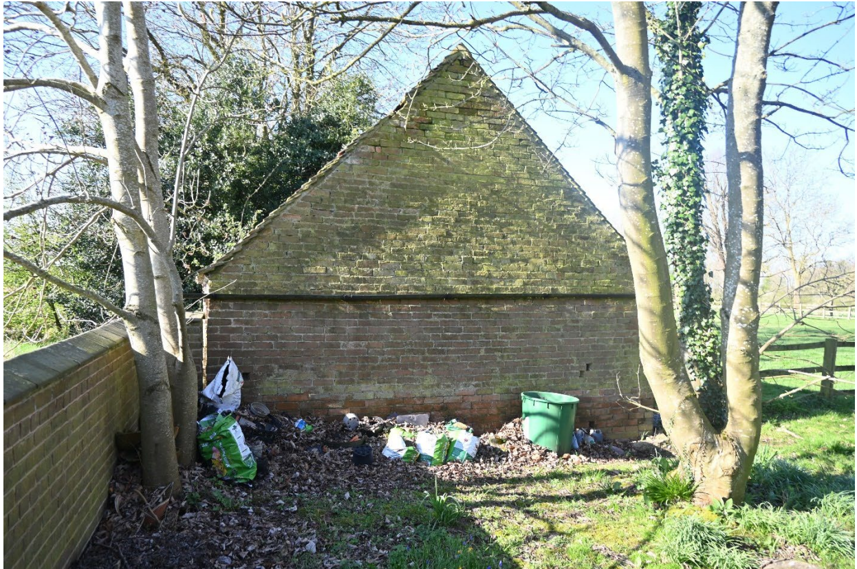
Fig. 6 Brick Stable and Boundary wall - Side View
