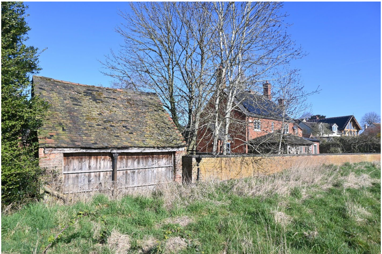
Fig. 7 Brick Stable and Boundary wall – Field View (rear)
