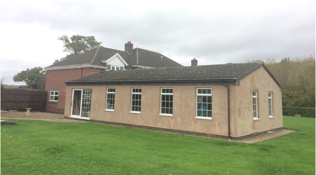
Image 3: Existing west elevation photo of existing pool room
