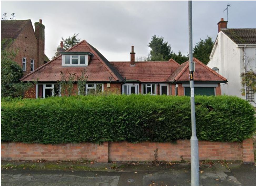
Fig. 6 Dormer Bungalow on Boyslade Road
