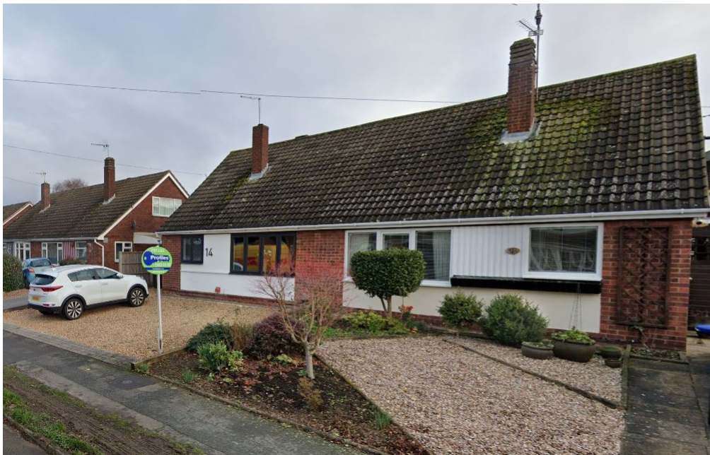
Fig. 9 1.5 storey dwellings along Boyslade Road
