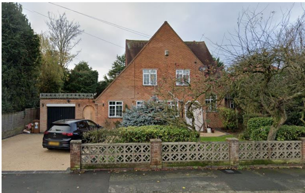
Fig. 7 Dormer Bungalow on Boyslade Road
