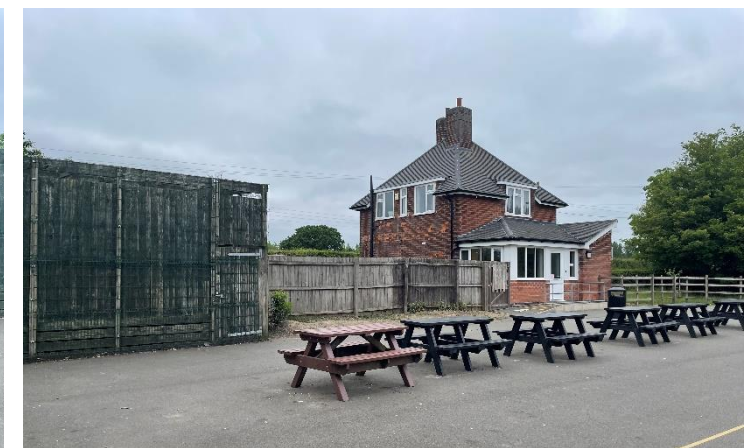
View from within the existing seating area looking towards the existing Learning Support unit.
