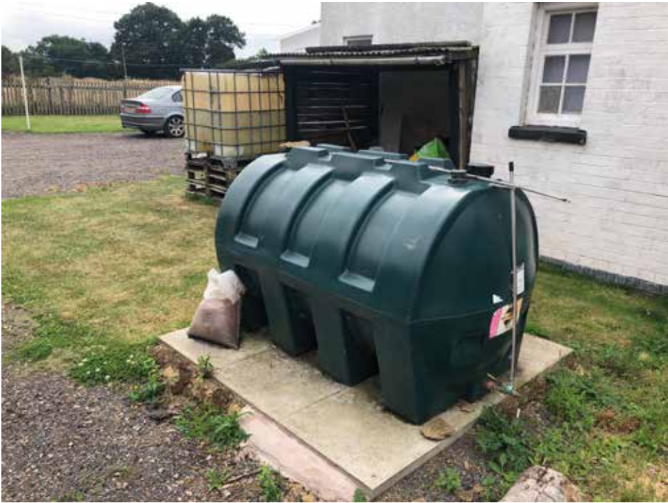
Oil storage tank at The Elms Farm
