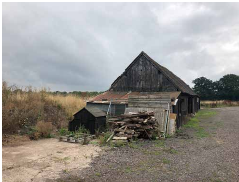
Rear of workshop buildings with earth mound
