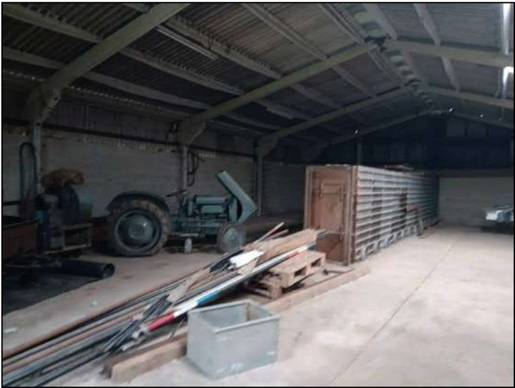
Photograph 6 – Inside Structure A
