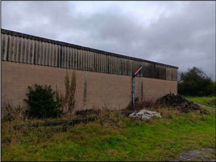
Photograph 7 – External Structure A
