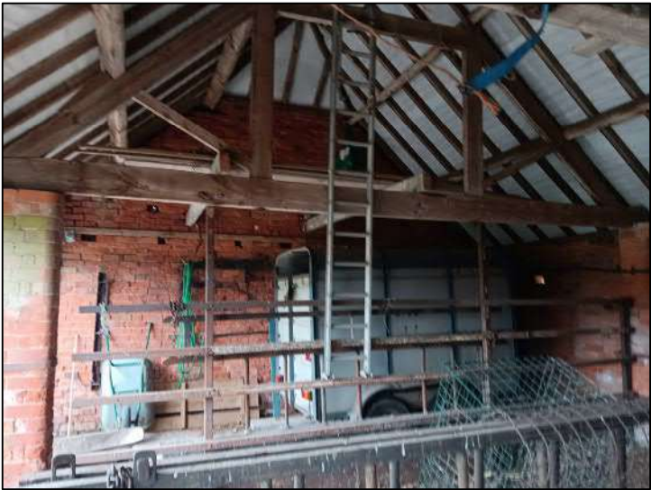
Photograph 18 – Structure E Internal
