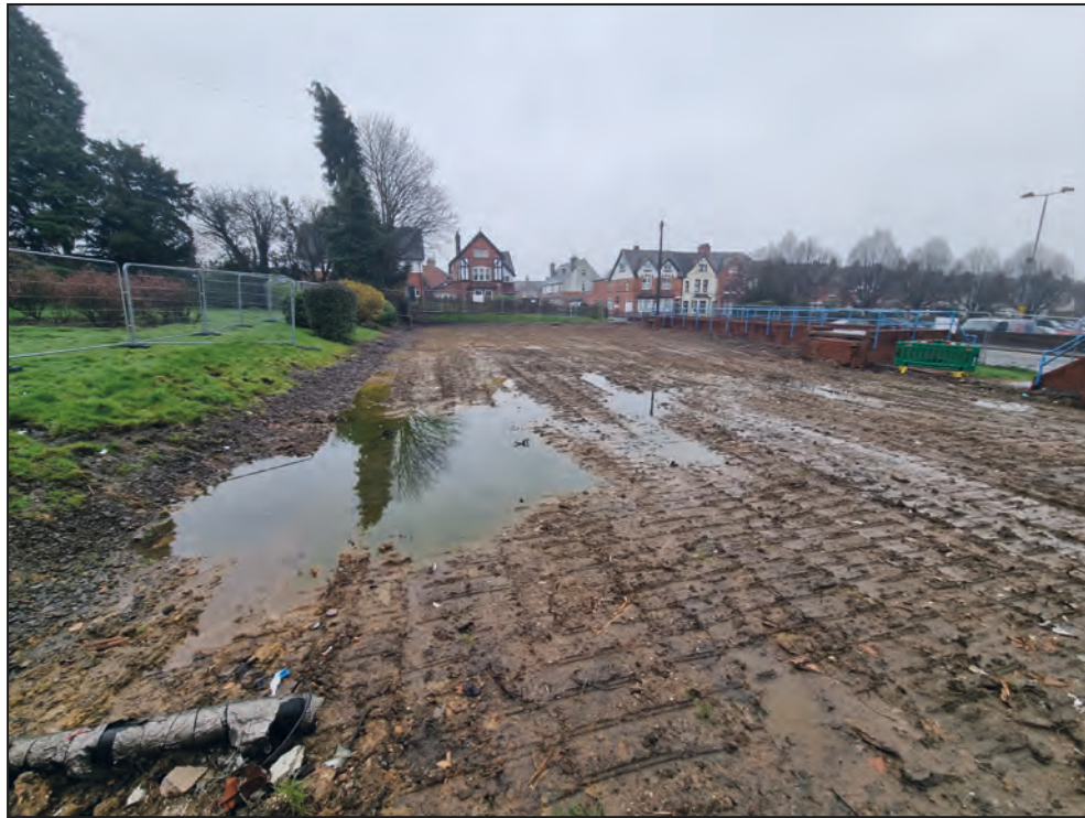
General view of Site, looking south-west
