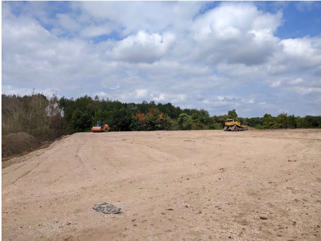
Photo 5: Further build up of Unit 2 levels achieved
