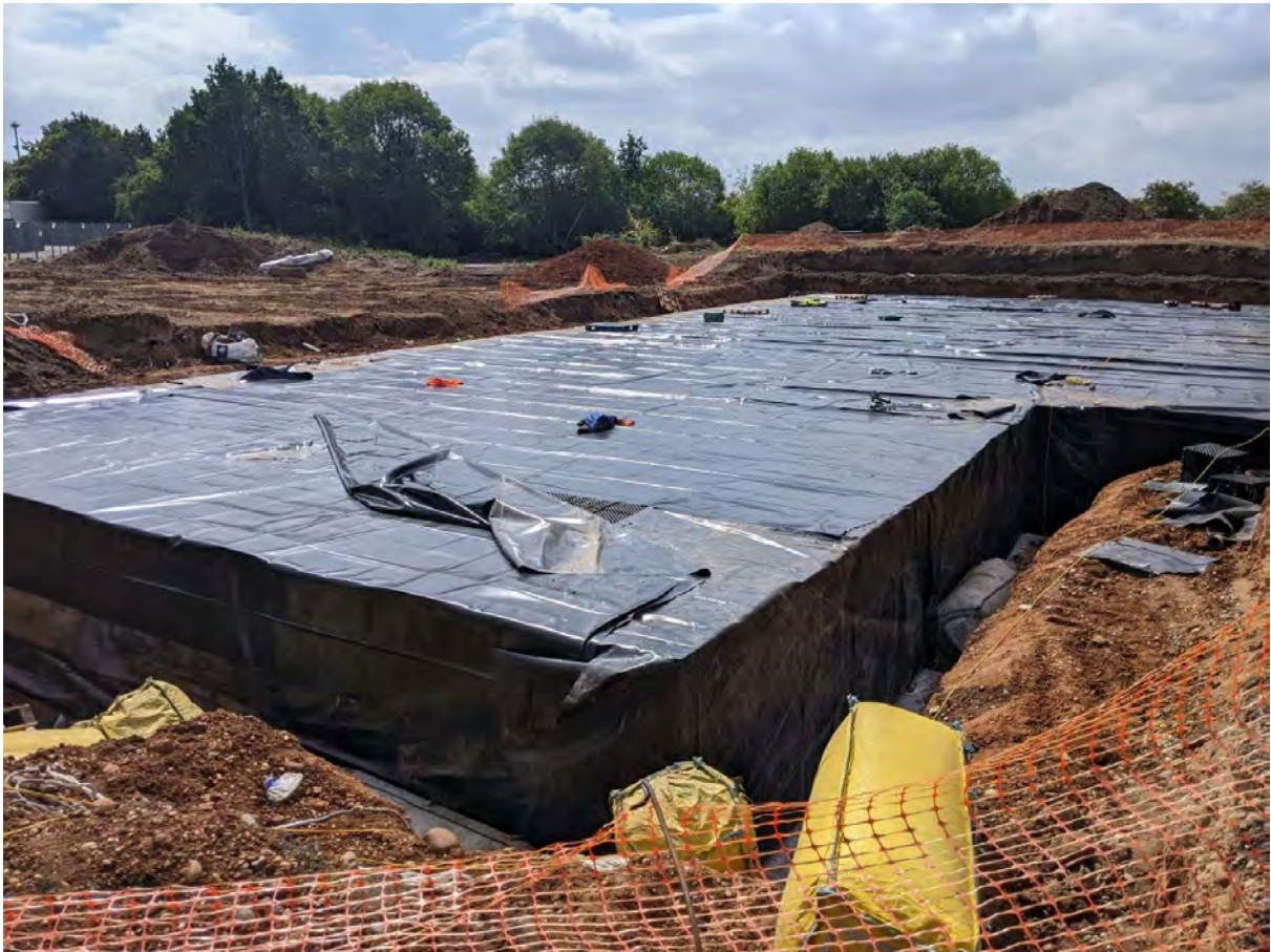
Photo 3: SW Attenuation tank area (south west of former badger sett)
