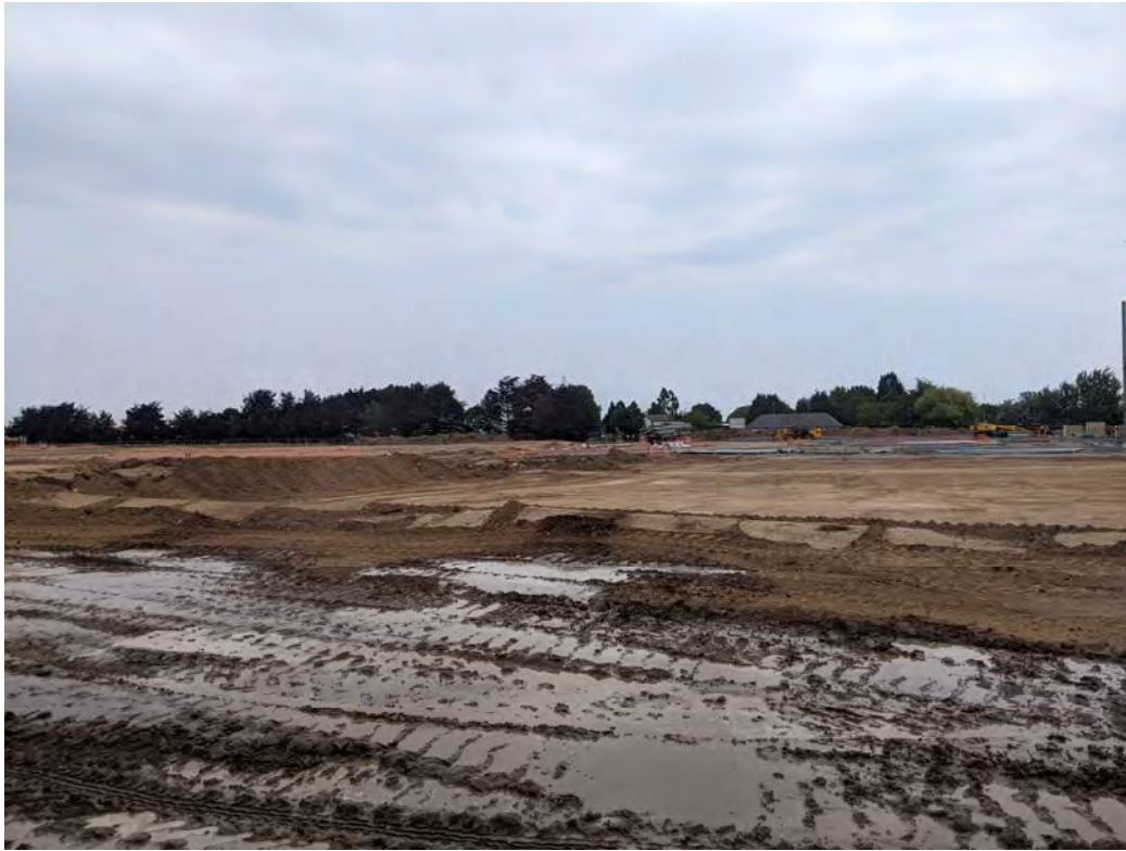
Photo 1: Initial strip of Phase 1 complete
