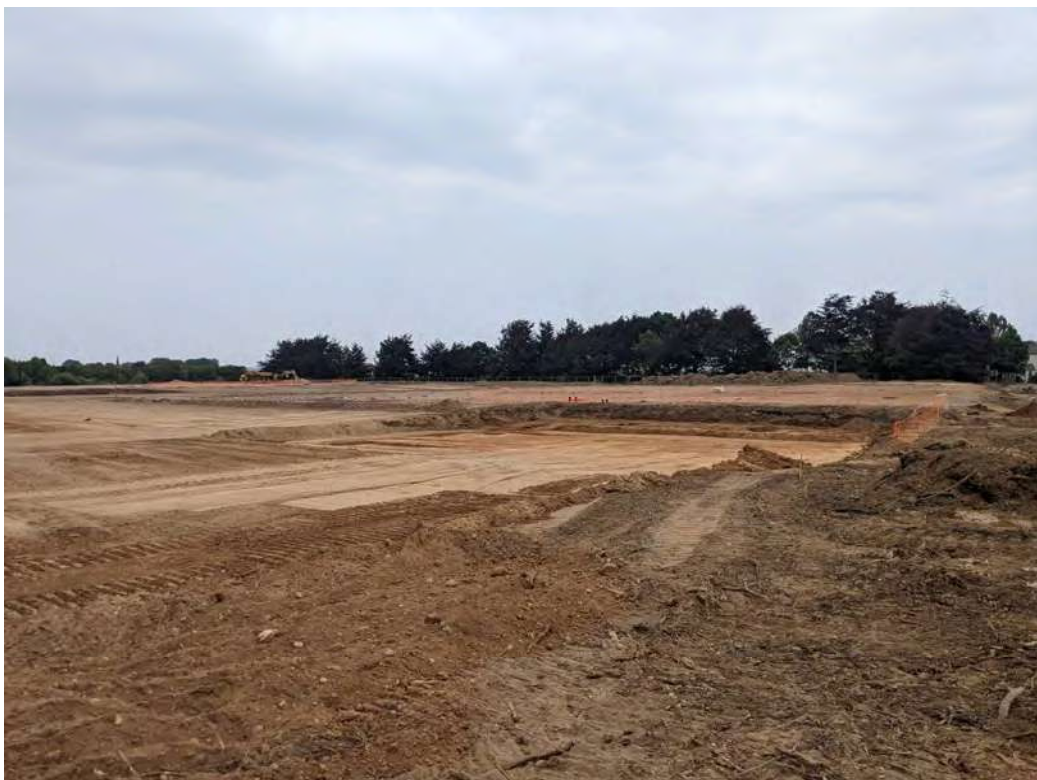
Photo 2: Strip and localised redistribution of materials across Unit 2 of Phase 1
