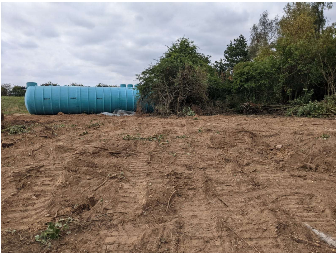
Photo 2: Former Badger Sett area looking north
