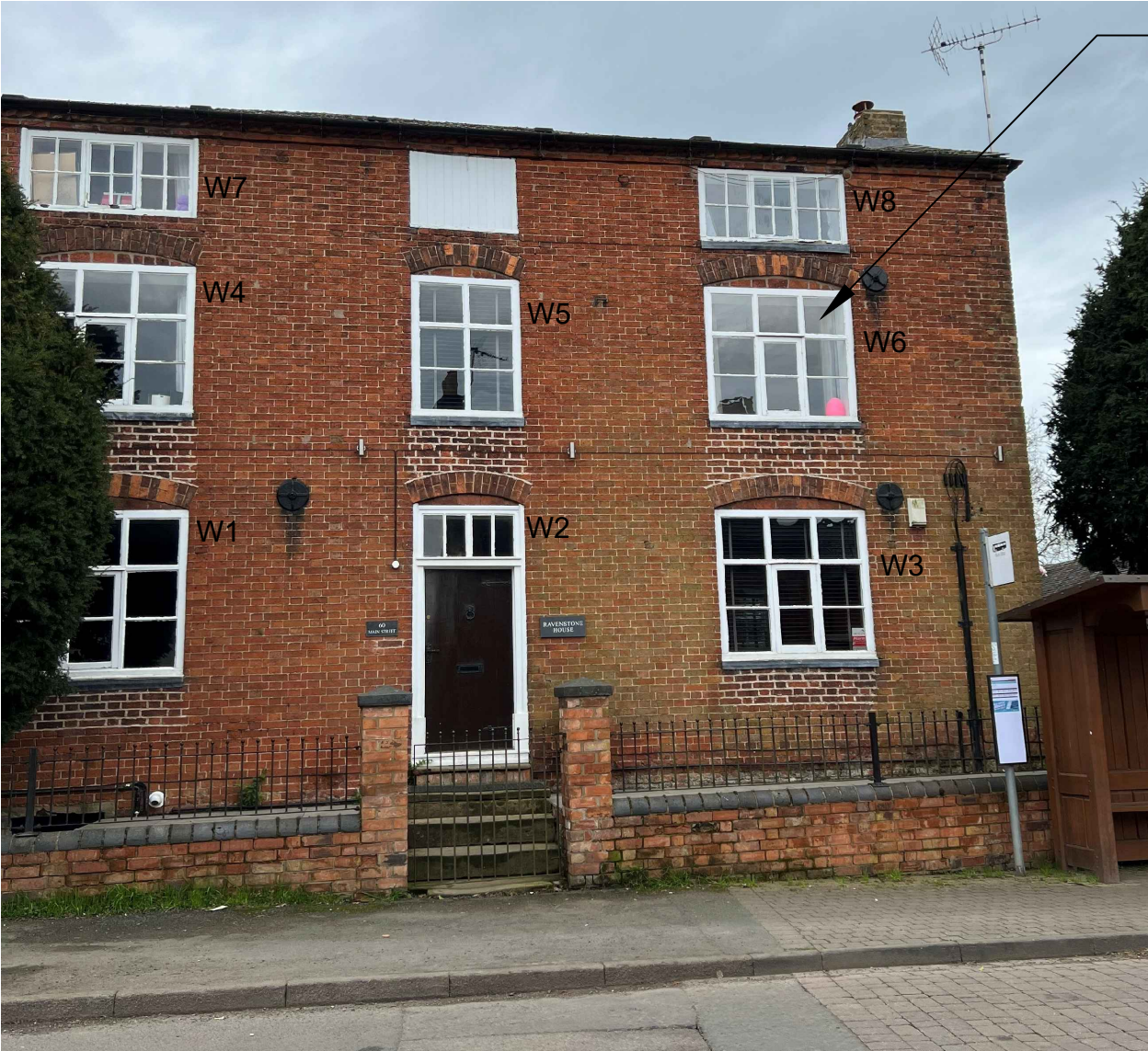
Window Replacement Front Elevation: W7, W8, Like For Like Replacement To Match The Existing Design, Size Material & Opening Type Front Elevation 8No. Windows To Be Replaced
