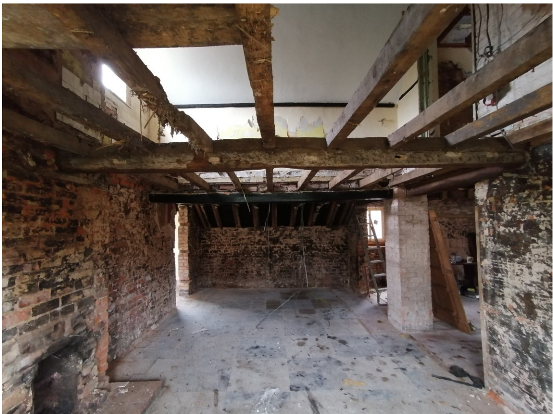
Plate 18; west-wing of former Moore's Arms showing re-used C17 wall-frame beam with mortices for square-panel framing.
