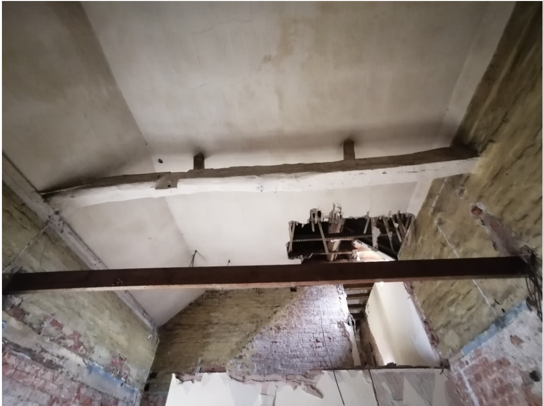
Plate 17; east wing of the former Moore's Arms showing possible re-used cruck.
