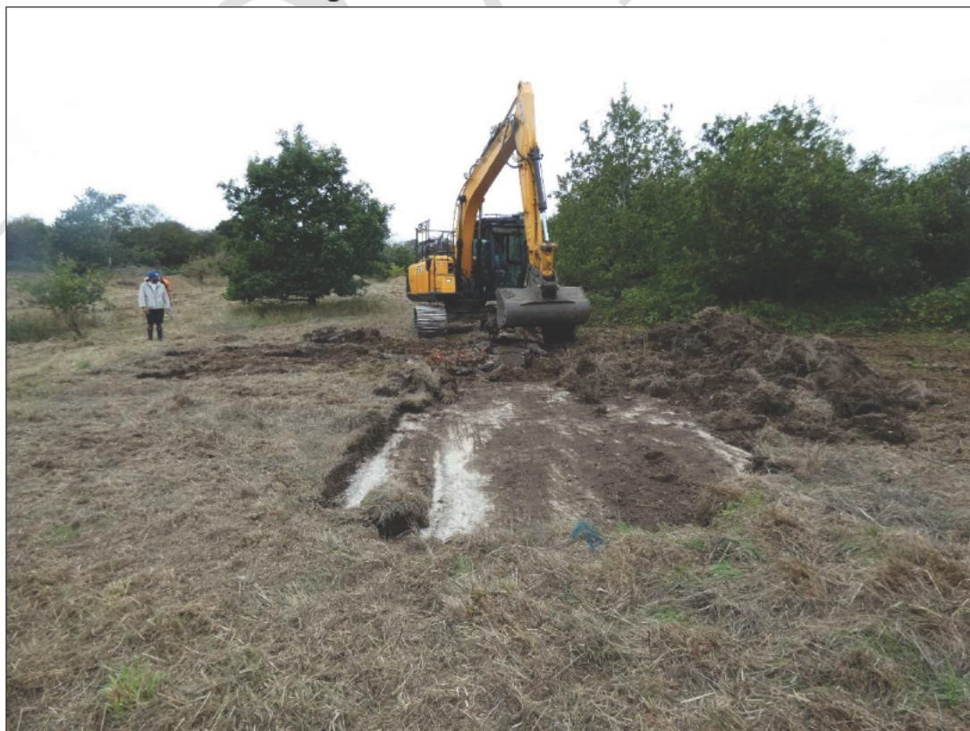
Figure 19: The concrete surface in the original location of Trench 15.
