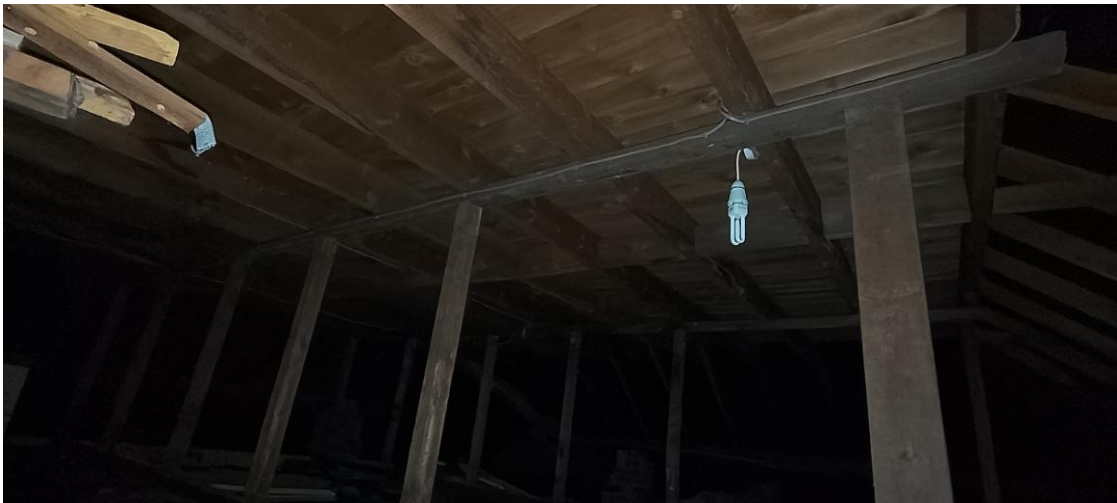
Plate 2: The accessible roof void showing the timber roof structure.
