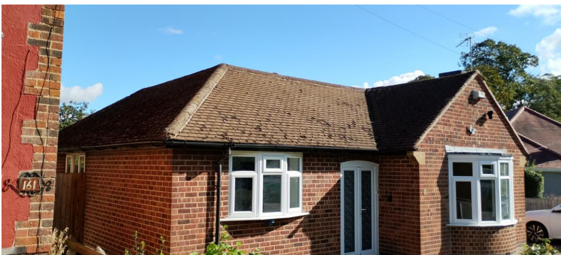
Plate 11: The front elevation and principal roof slopes of the main dwelling.
