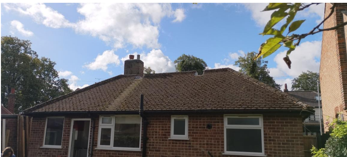
Plate 5: The rear elevation of the main dwelling and tiled roof.
