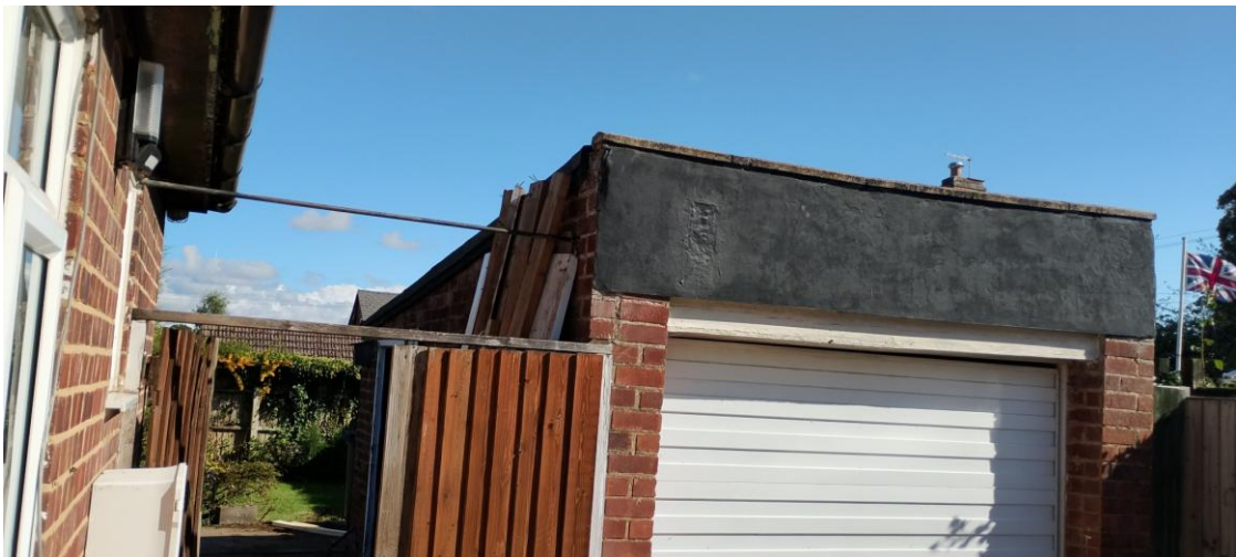
Plate 13: A close view of the garage eaves and roof junction.
