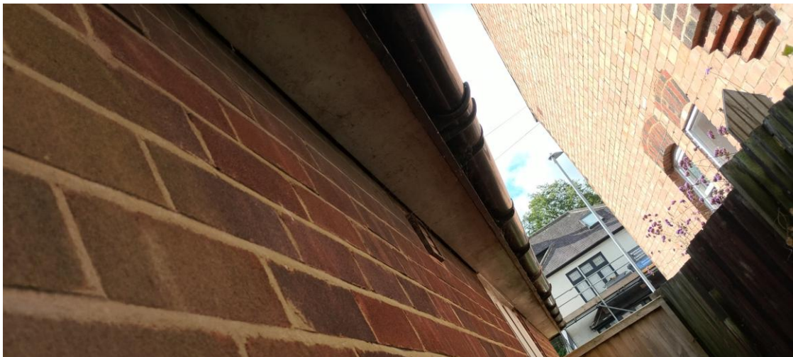
Plate 7: A close view of the eaves and wall junction between the dwelling and neighbouring building.
