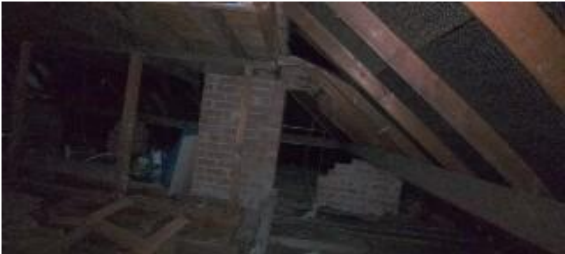
Plate 4: An overview of the roof void and chimney breast.
