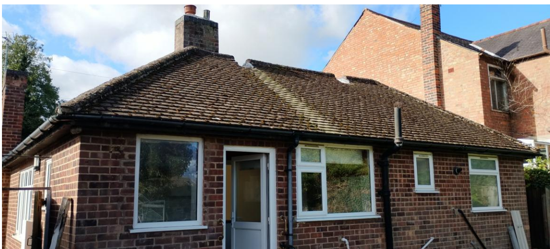
Plate 8: The main dwelling viewed from the garden, showing its brick elevations and pitched tiled roof.
