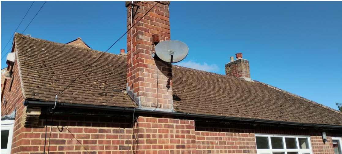
Plate 10: The side roof slope, chimney, eaves and associated rainwater goods.
