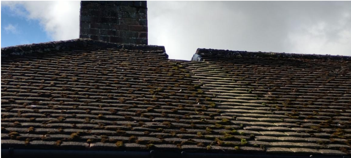
Plate 9: A close view of the tiled roof covering and chimney.
