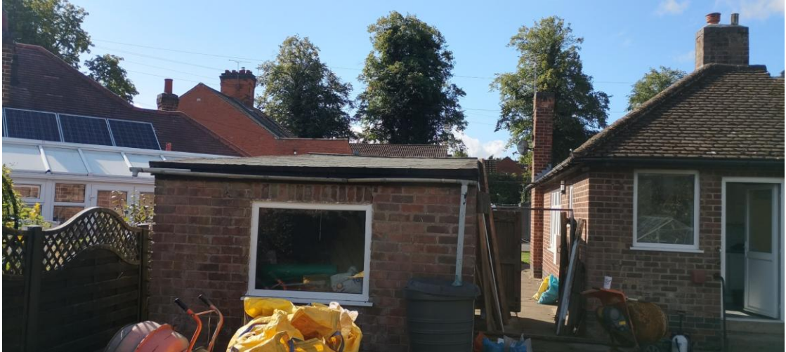
Plate 15: The detached garage viewed from the rear garden, with the main dwelling beyond.
