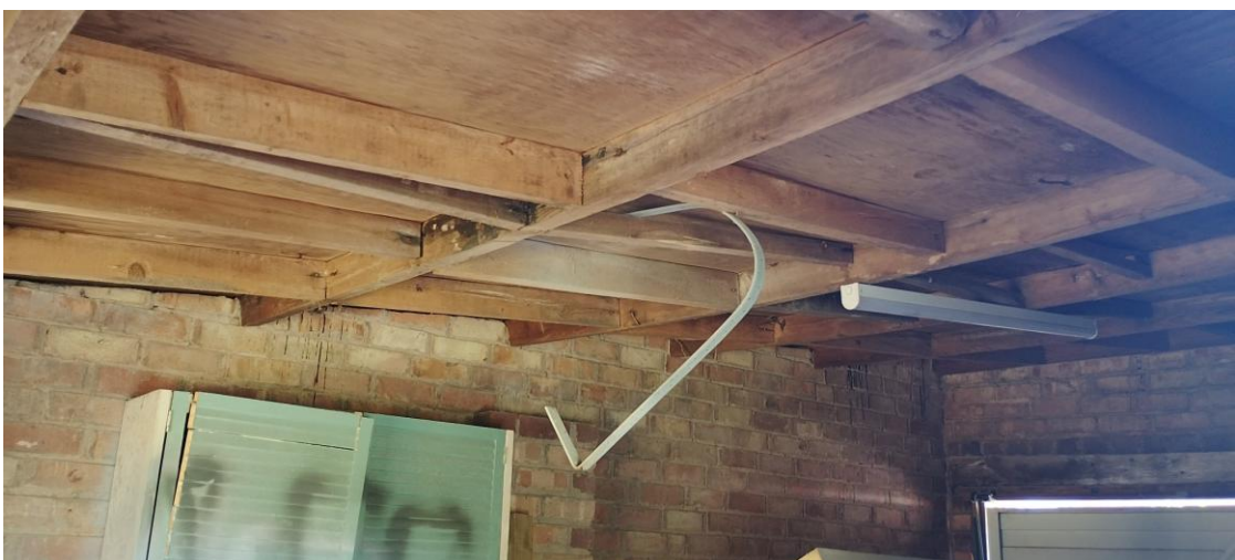
Plate 14: The internal structure of the detached garage roof.
