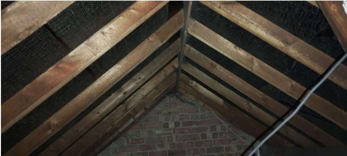
Plate 3: The internal roof structure and brick gable wall.
