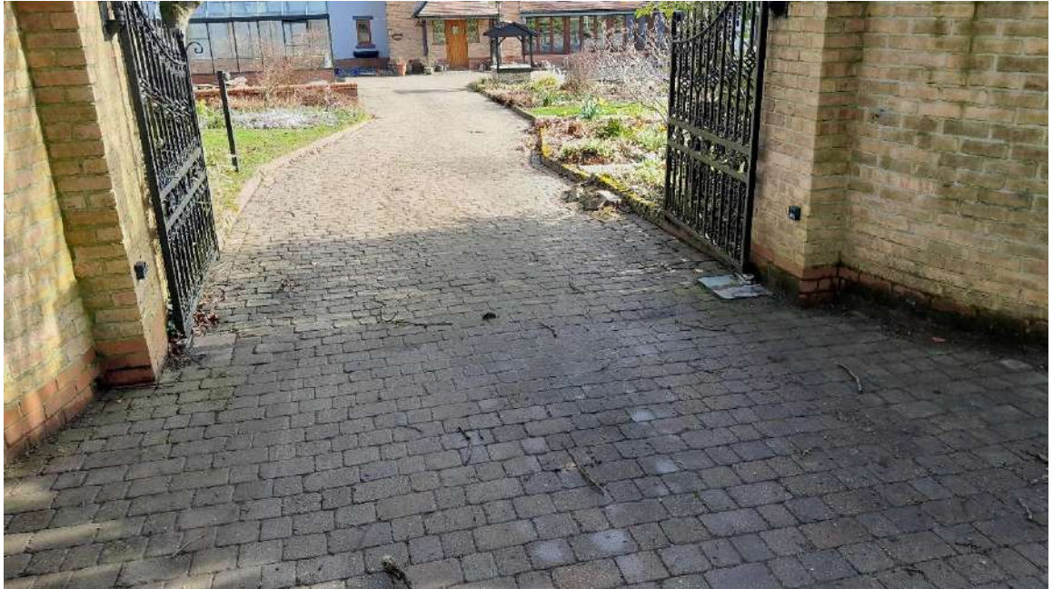
Plate 1 – Sealed hardstanding driveway
