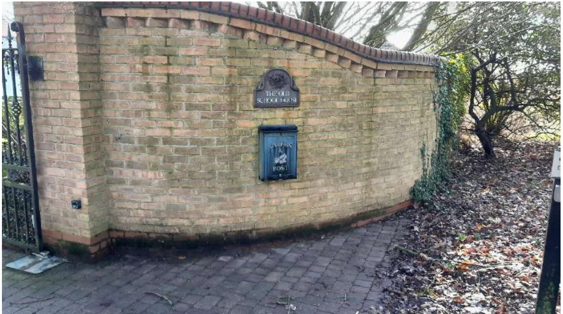
Plate 2 – Impermeable brick-built wall
