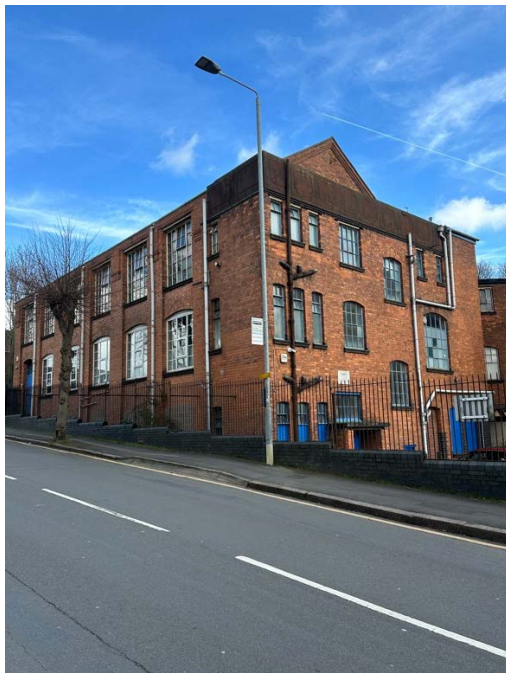
Site photos of View from Council Road.
