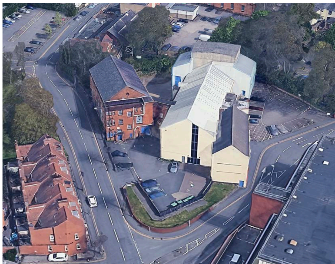
Aerial View of Concordia Theatre from Stockwell Head with service area in prominent location
