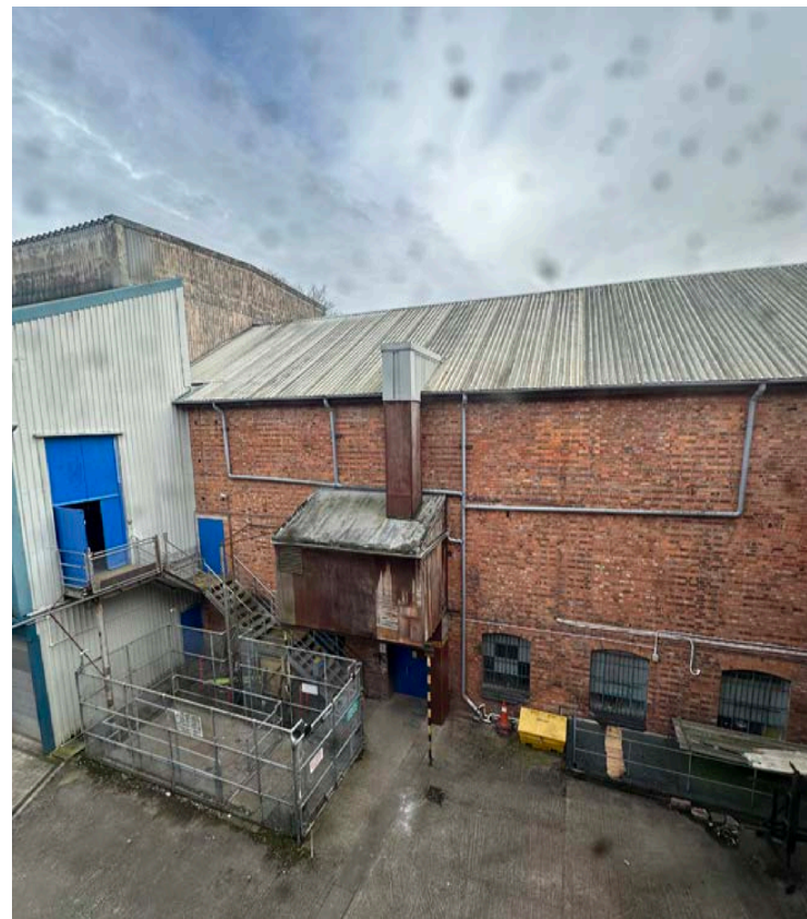
Flytower, Scene Lift, HVAC and Auditorium Roof
