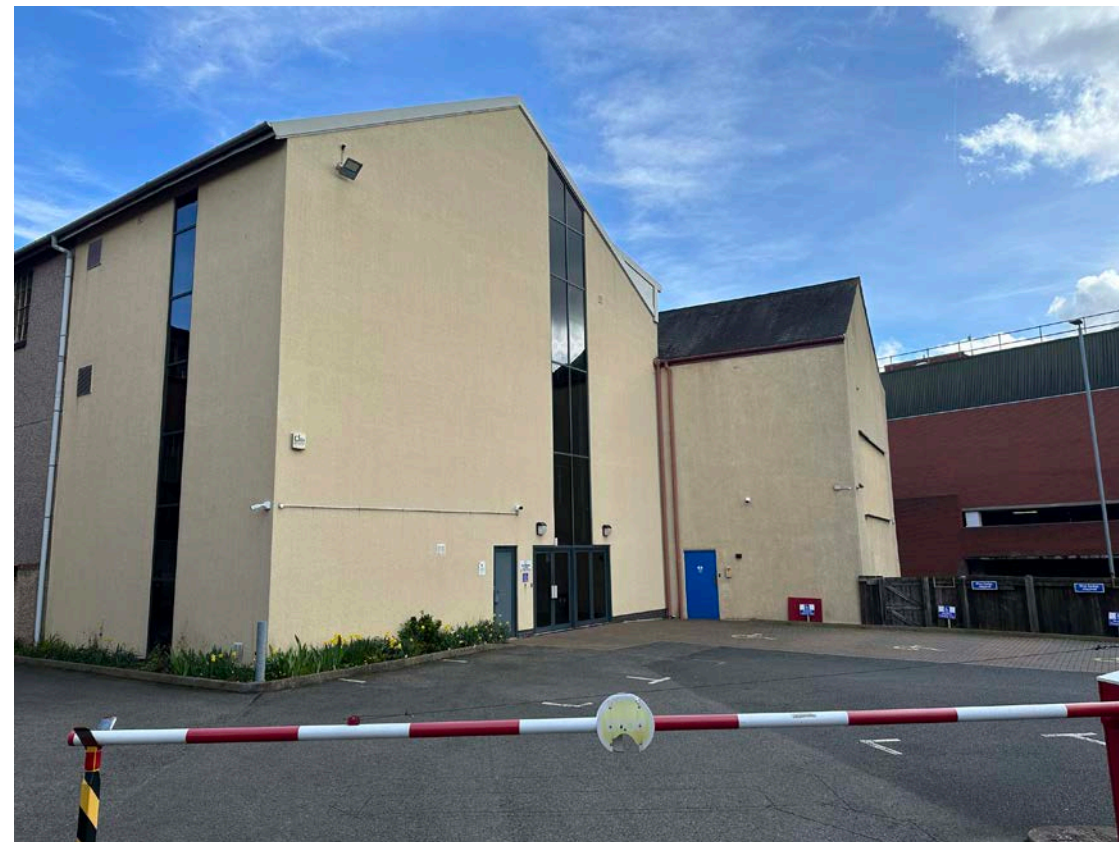
Service Yard and Disabled Persons Entrance
