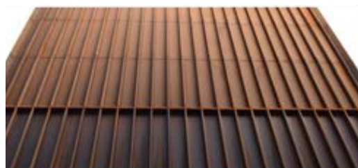
Ribbed metal panelling at Hallé Orchestra Manchester
