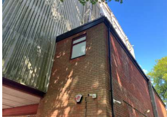
Photograph 2: fascia boarding of single-storey extension of B1
