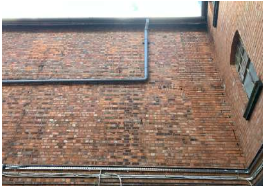
Photograph 3: missing mortar on west elevation of B1
