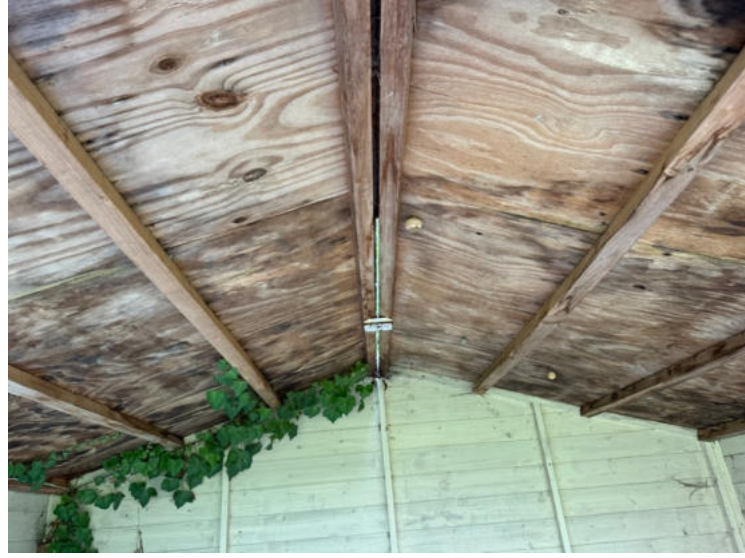
Photo 6: Building B2 interior
