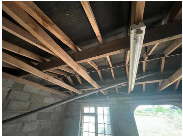
Photo 12: Building B1 interior
