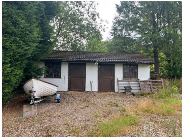
Photo 8: Building B1 exterior
