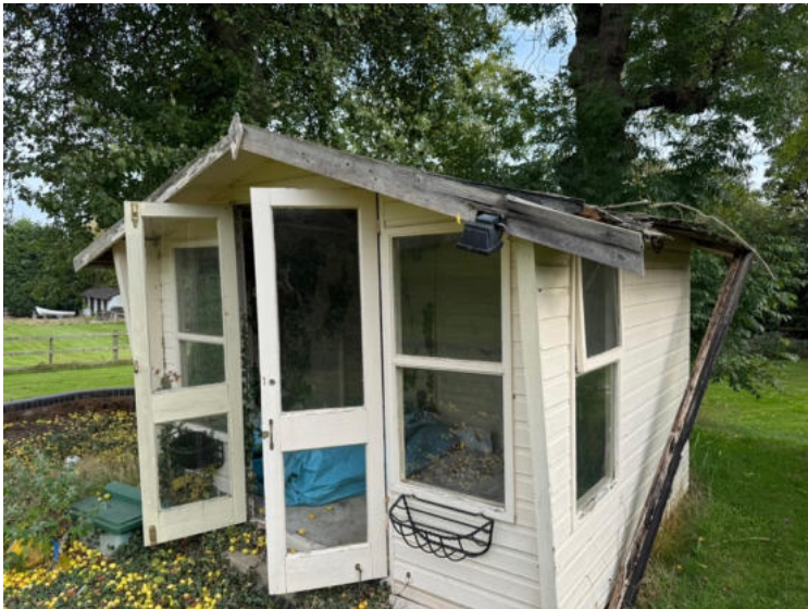
Photo 7: Building B2 exterior
