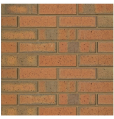
Brickwork to chimney lbstock Etruria mixtture
