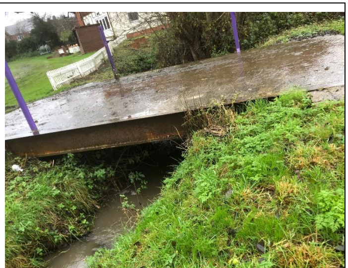
FIGURE 2: FIRST PEDESTRIAN CROSSING APPROXIMATELY 25M UPSTREAM OF SITE
