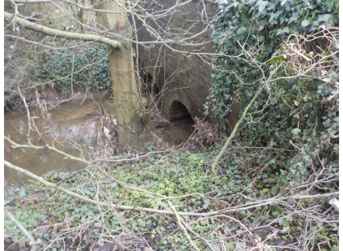
FIGURE 12: DOUBLE ARCH CROSSING AT DESFORD LANE
