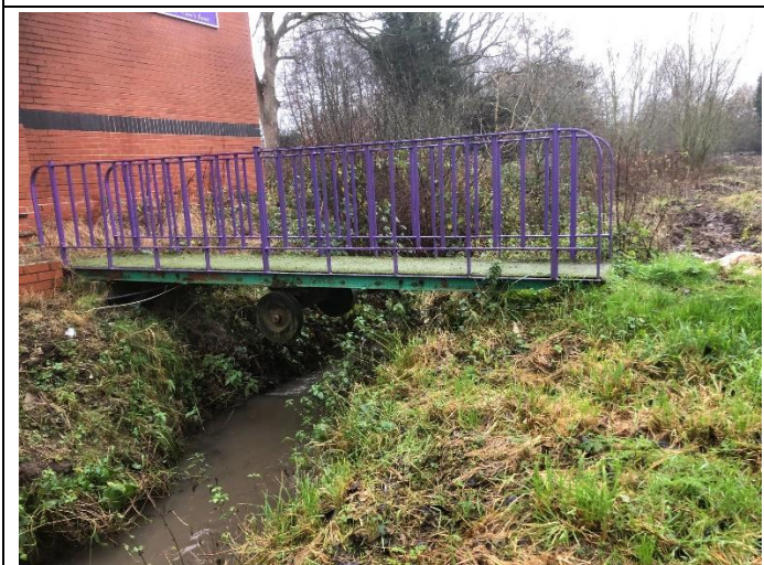
FIGURE 3: SECOND PEDESTRIAN CROSSING ADJACENT TO THE SITE.
