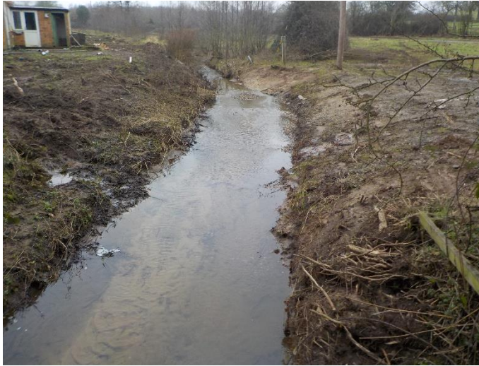
FIGURE 11: UPSTREAM SECTION OF THE WATERCOURSE, BEFORE DOUBLE ARCH CULVERT
