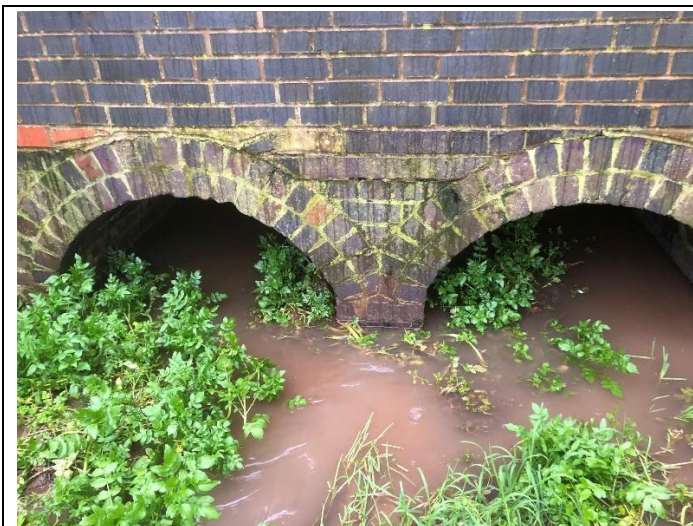
FIGURE 1: WATERCOURSE PASSING UNDERNEATH DESFORD LANE VIA A DOUBLE ARCH CULVERT, 250M UPSTREAM OF DEVELOPMENT SITE
