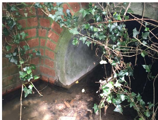
Photo 12: View of Surface Water Sewer entering land drain in south west corner of Field 4
