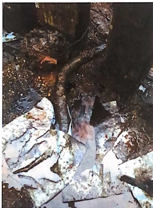
Plate 4: Free phase heating oil within the excavation
