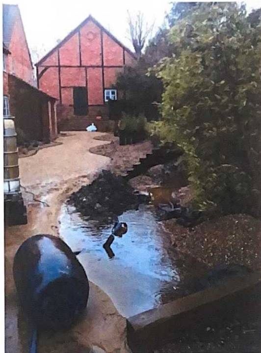
Plate 3: Free phase oil on the surface of the standing water within the affected area
