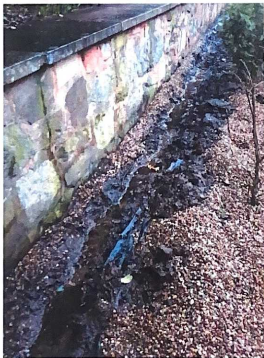
Plate 2: Trench excavated by the insured following the discovery of the escape of oil
