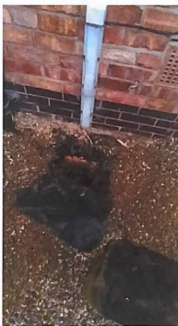
Plate 6: Small trench advanced next to the house showing free phase oil above the footing
