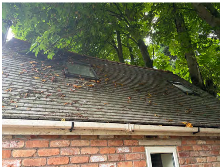
Image 3 - Northern elevation of B1, and general condition of roof tiles.
