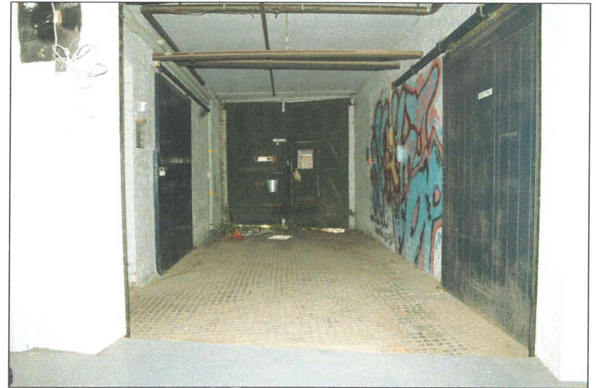
Inside of goods entrance. Looking east.
