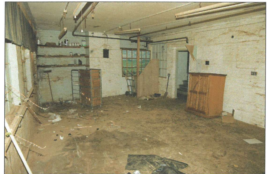
Main building, ground floor. Blocked windows on rear wall and inserted doorway. Looking south-west.
