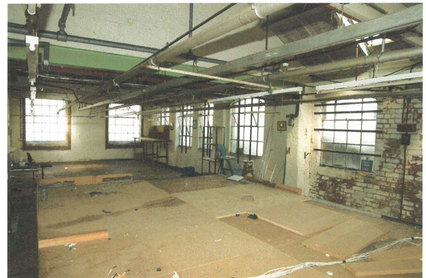
Gable-ended building, first floor. Blocked remnant of rear Venetian windows in gable. Looking north-east.
