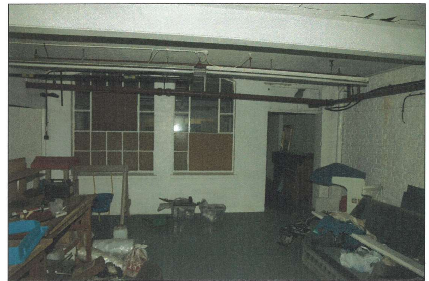
Gable-ended building, ground floor. Original back wall and windows. Looking east.
