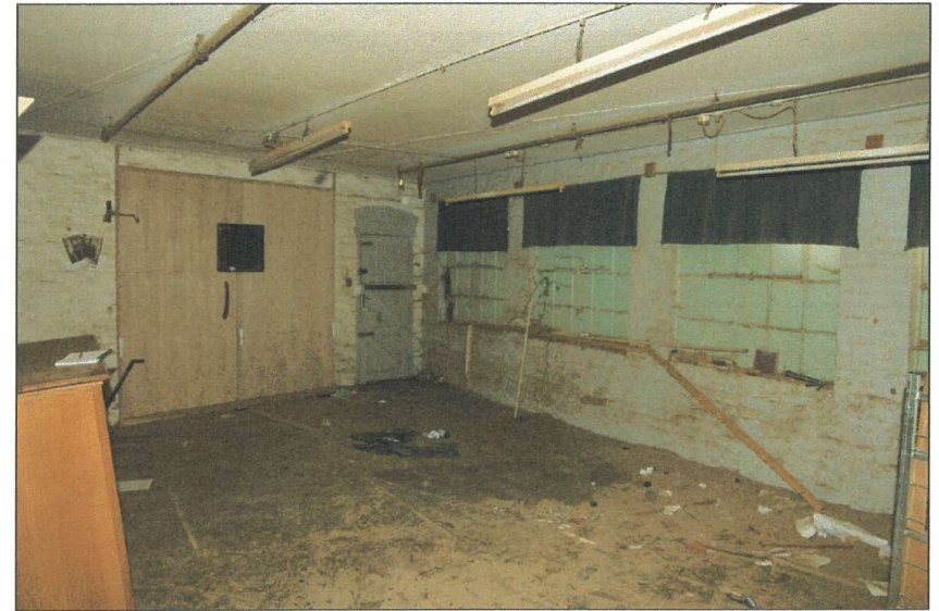
Main building, ground floor. Front windows and north wall. Looking north-east.
