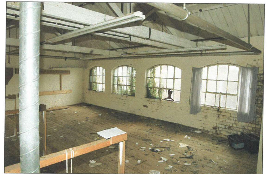
Main building, first floor. Front windows. Looking north-east.
